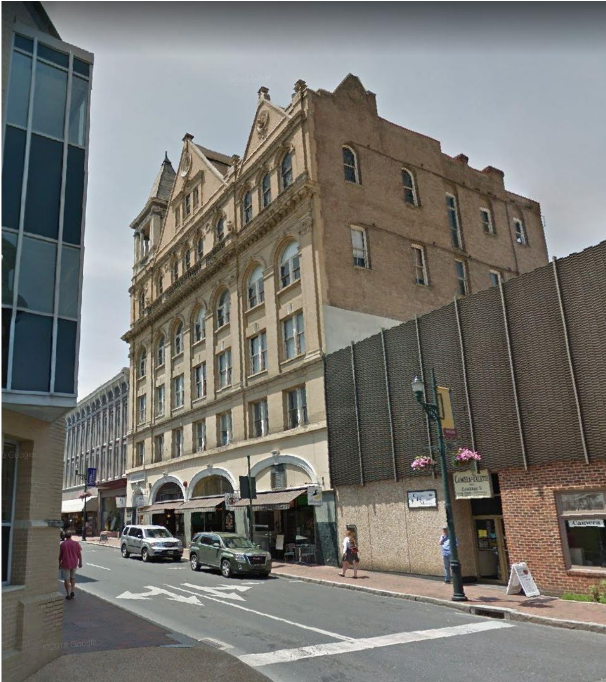
13 West Beverley Street – 5½ stories with roof belvedere
