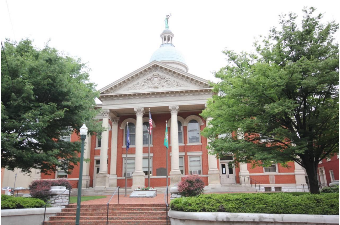
1 East Johnson Street
