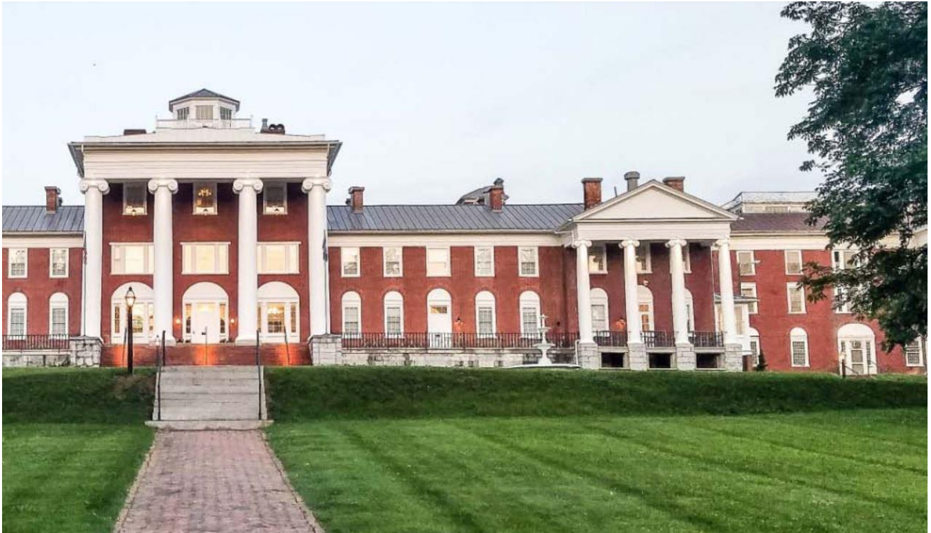
The Blackburn Inn – 3 stories with tower, 3 and 4 stories
