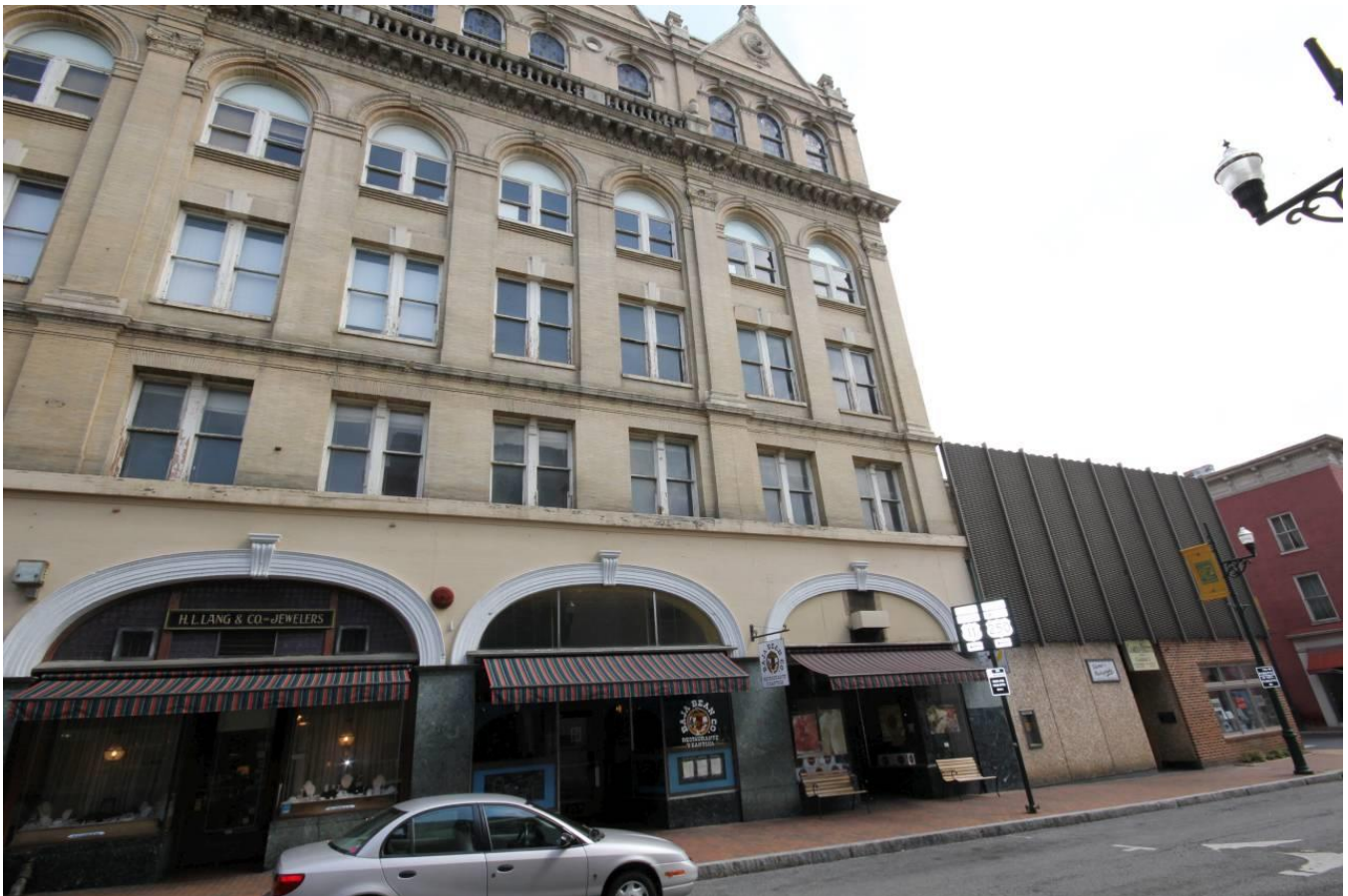
13 West Beverley Street – 5½ stories with roof belvedere
