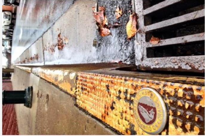
Storm drain in downtown Staunton
