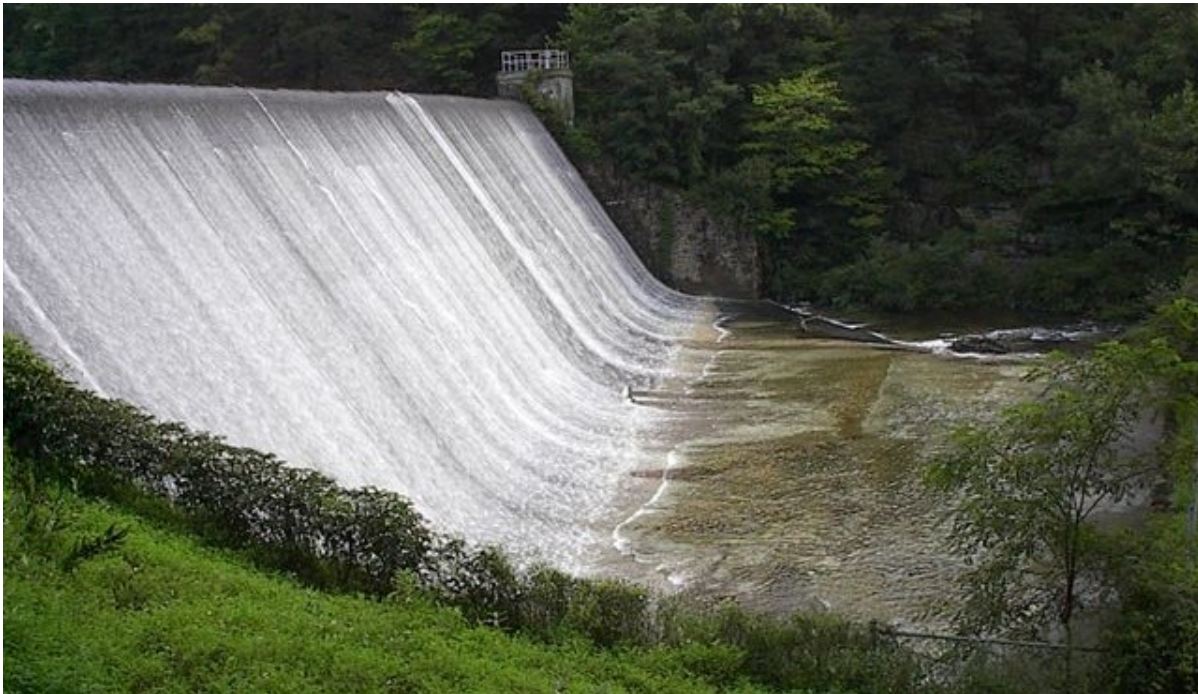
Staunton Dam - One of the City's water sources
