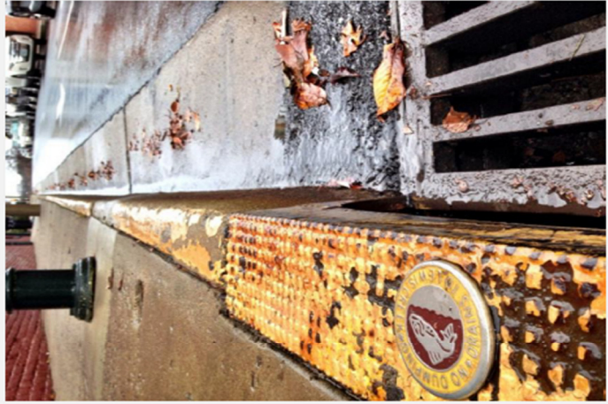
Storm drain in downtown Staunton
