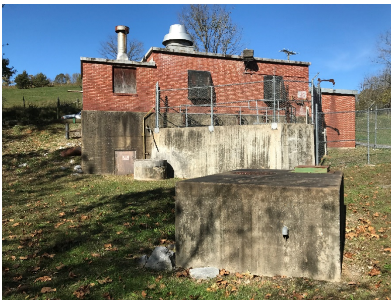
Figure 2.2: Existing Gardner Spring Pump Station
