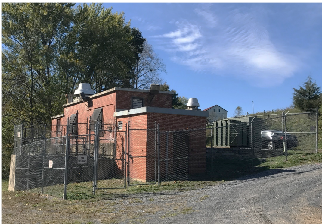
Figure 5.4: Existing Gardner Spring Pump Station Site
