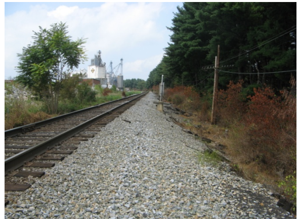
CSX Railroad Along Southwestern Boundary
