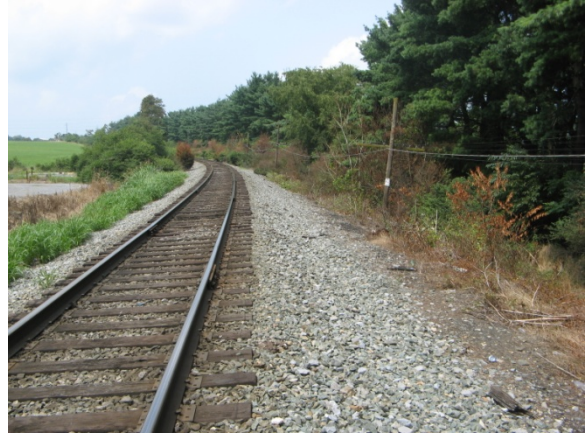
CSX Railroad Along Southwestern Boundary
