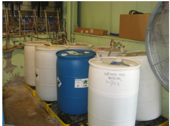
Detergent Storage in Laundry
