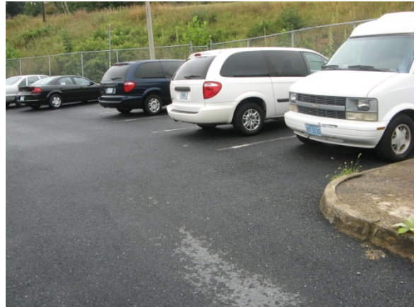
Location of USTs at Physical Plant Services/Materials Management Building
