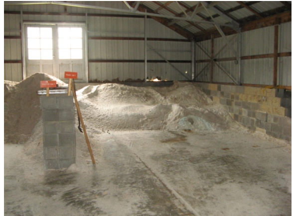
Salt Storage at WWTP Site
