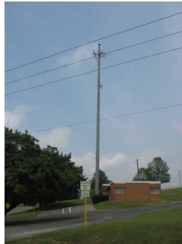
Call Tower at State Police Refueling Station
