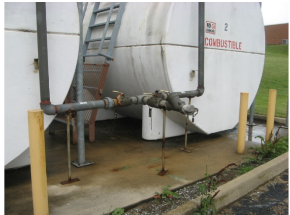
Fill Port of ASTs at Power Plant
