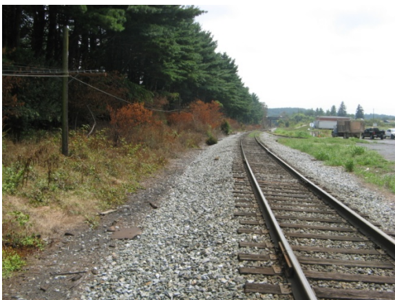
CSX Railroad Along Southwestern Boundary
