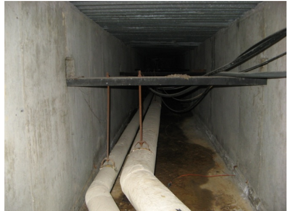
Steam Tunnel at Building 127
