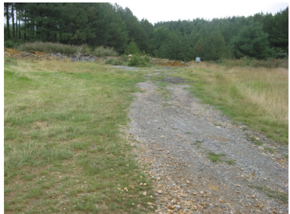
Fill Area North of WWTP Site
