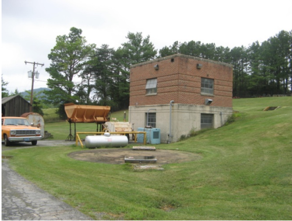
WWTP Pump Station
