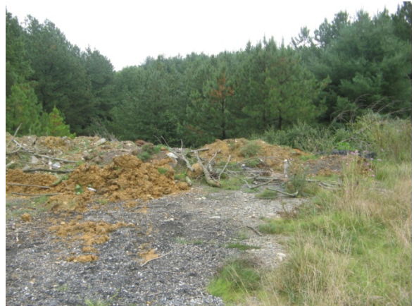
Fill Area North of WWTP Site
