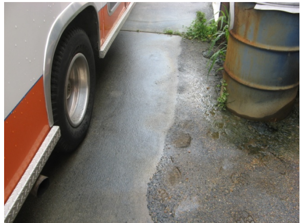
Oily Sheen on Asphalt at Waste Fluid Storage Outside of Physical Plant Services/Materials Management Building
