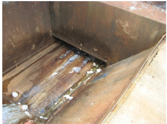
Compactor at WWTP Site
