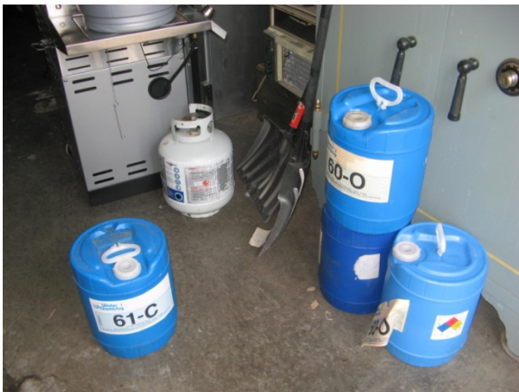
Boiler Water Chemicals in Physical Plant Services/Materials Management Building
