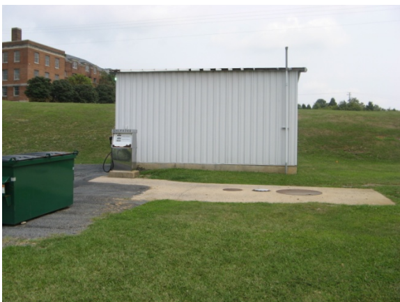
UST at State Police Fueling Station
