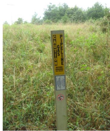
Natural Gas Pipeline Crossing Northeast Corner of WSH Property
