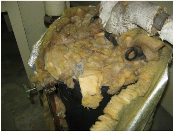
Pipe Insulation in Building 127
