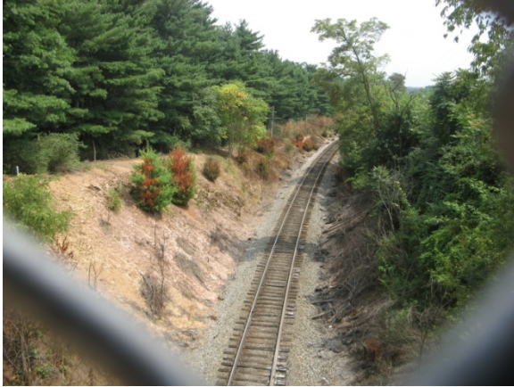
CSX Railroad at Frontier Drive
