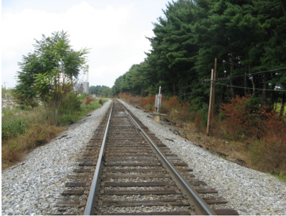
CSX Railroad Along Southwestern Boundary
