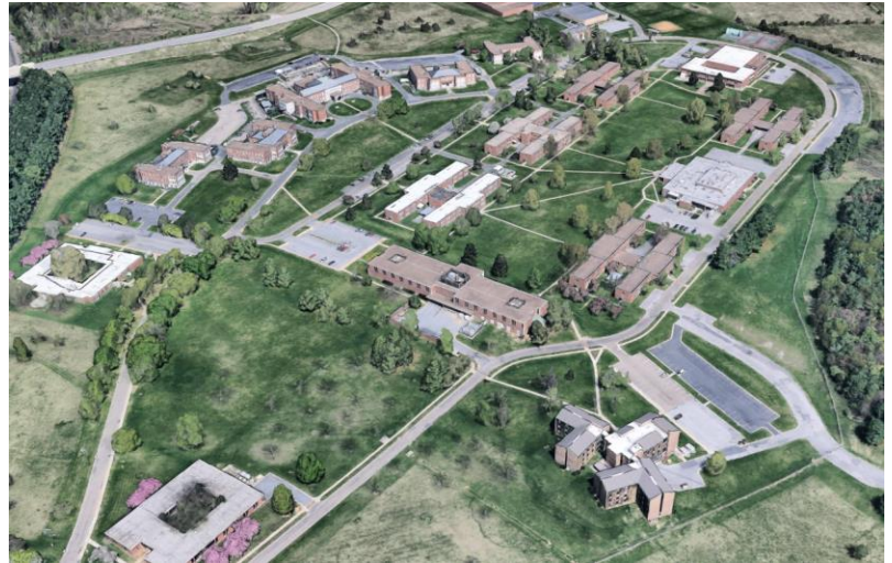
Demolition offers a significant public relations and marketing opportunity.
