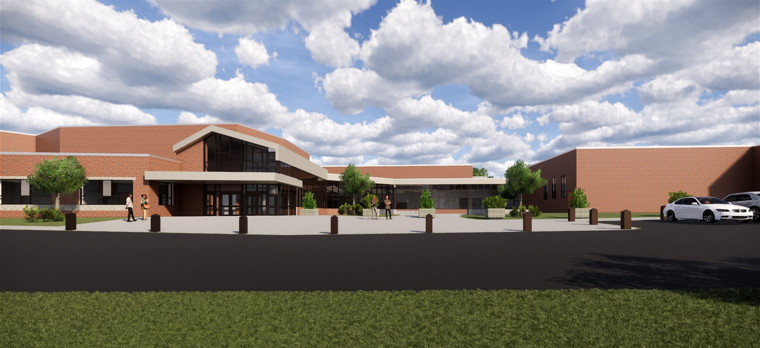
STAUNTON HIGH SCHOOL – CONSTRUCTION PROGRESS UPDATE SEPTEMBER 9, 2019
