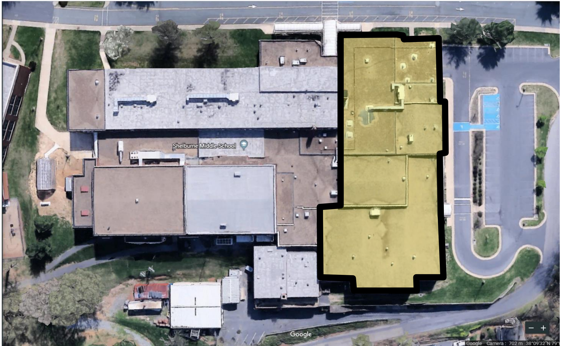
AERIAL VIEW OF SHELBURNE MIDDLE SCHOOL With Highlighted Roof Section to be Treated (Estimated 36,692 Square Feet)
