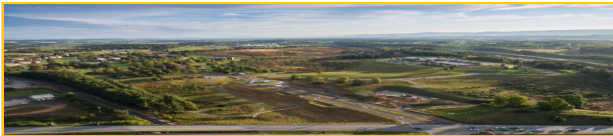
Staunton Crossing Development Site
