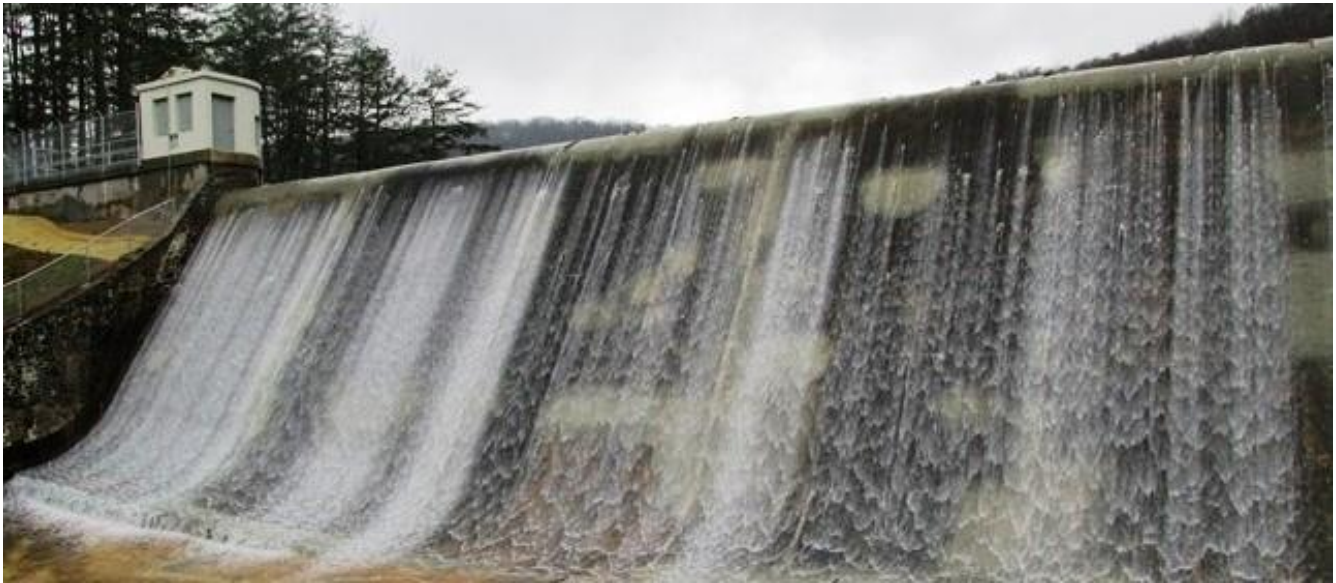
Dam at Staunton Reservoir - One of the City's water sources
