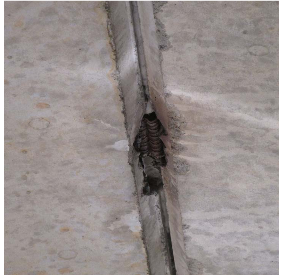
Photo 6 - Close-up view of the joint between two adjacent precast concrete single tees. We noted the joint connecting the adjacent tees consisted of a piece of steel reinforcement welded to a partially exposed piece of reinforcement embedded into the edge of each of the adjacent tees.
