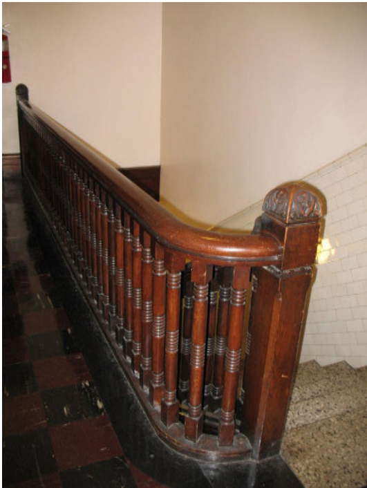
Detail of original second floor decorative guardrail at the top of the stair.
