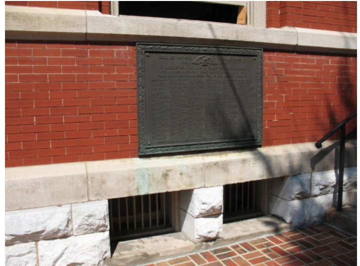
View of rusticated native limestone foundation and dressed Indiana limestone water table.
