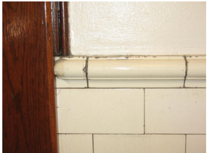
Detail of plaster, ceramic tile wainscot and wood trim in first floor corridor.
