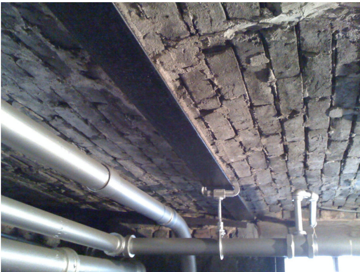
Photo #1: Existing beam and brick vault floor structure.
