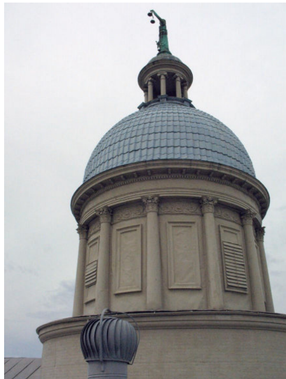
View of cupola showing decorative sheet metal work, ribbed metal shingle roof and bronze statue.
