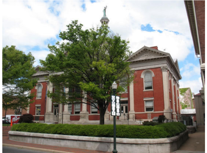
View of courthouse from E. Johnson Street showing sidewalk and retaining wall.
