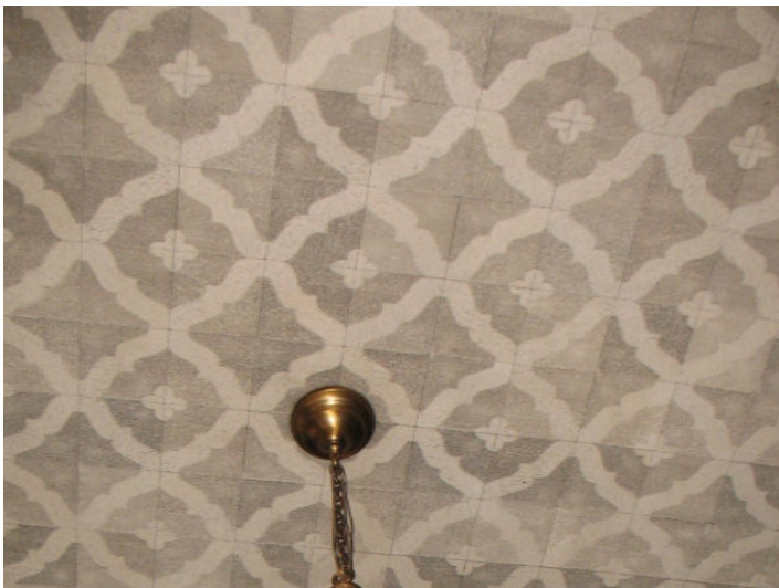
Acoustical ceiling tiles installed during 1949 courtroom renovation.
