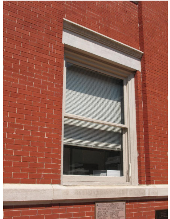
Detail of original first floor window.
