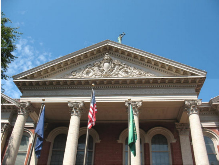
Photo of pediment above front portico showing decorative sheet metal cornices.
