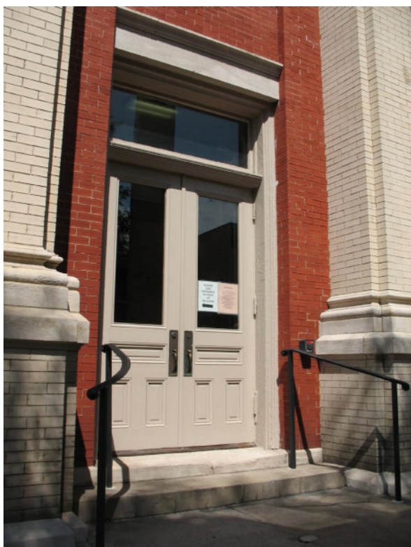
Original entrance into hyphen directly adjacent to front portico.
