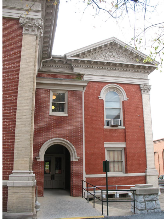
The existing concrete handicap ramp leads from Barristers Row Alley to the northwestern entrance to the courthouse.
