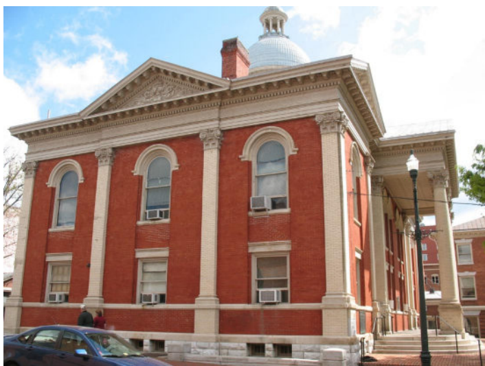
The west elevation of the courthouse faces South Augusta Street.
