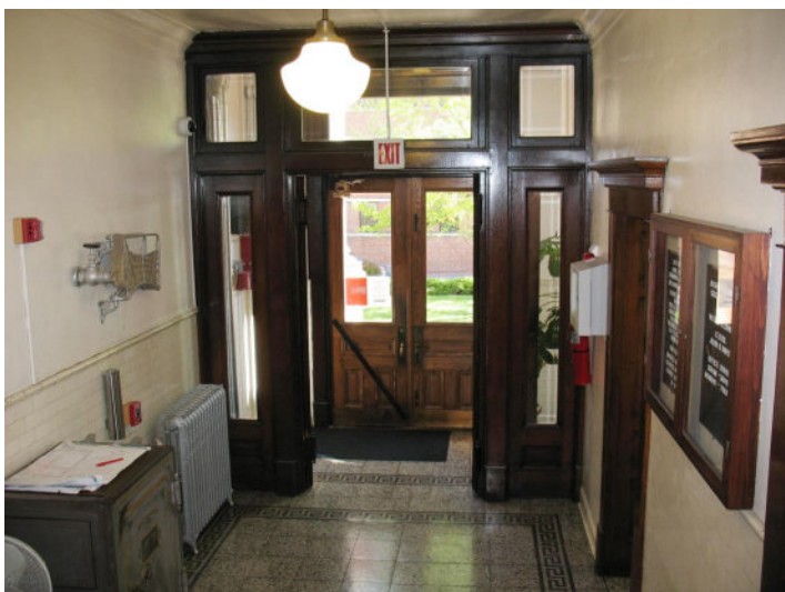
East corridor looking south through vestibule.
