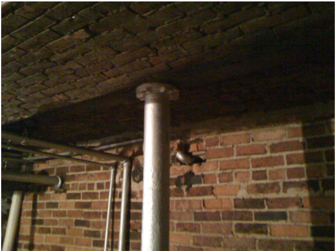
Photo #3: Shoring post located beneath existing beam in basement ceiling
