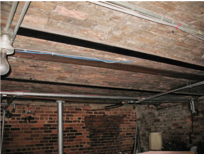
View of first floor brick vault floor structure as seen in the basement.
