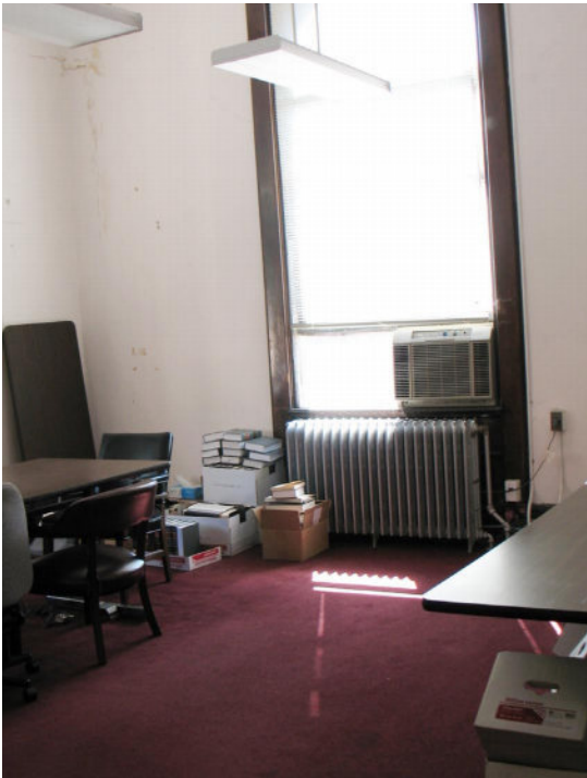
Carpet has been installed over the original floors in several locations.
