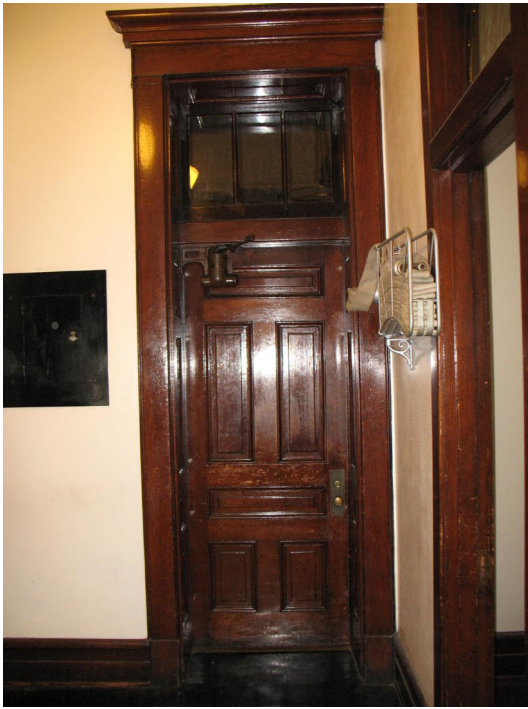
Typical door with transom and header cap on second floor.
