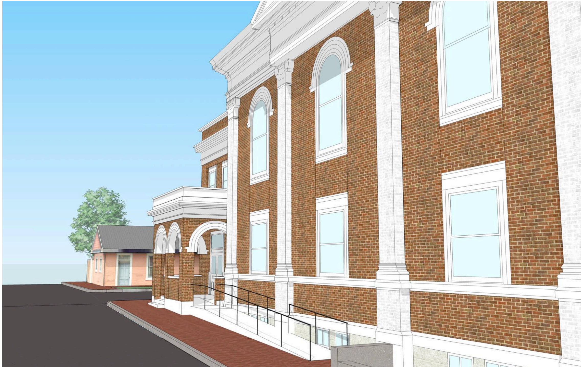
Looking north at the Augusta Street elevation, the new handicap ramp provides access from the sidewalk at the side of the building to the new main entrance.
