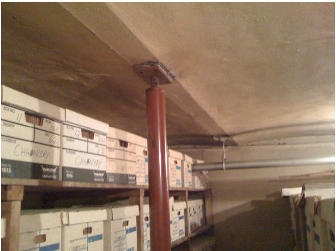
Photo #4: Adjustable steel column shoring post under steel beam supporting HD files above
