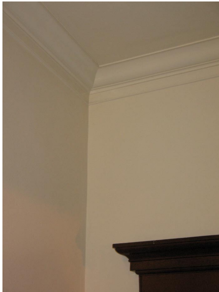
Detail of plaster crown molding in first floor corridor.
