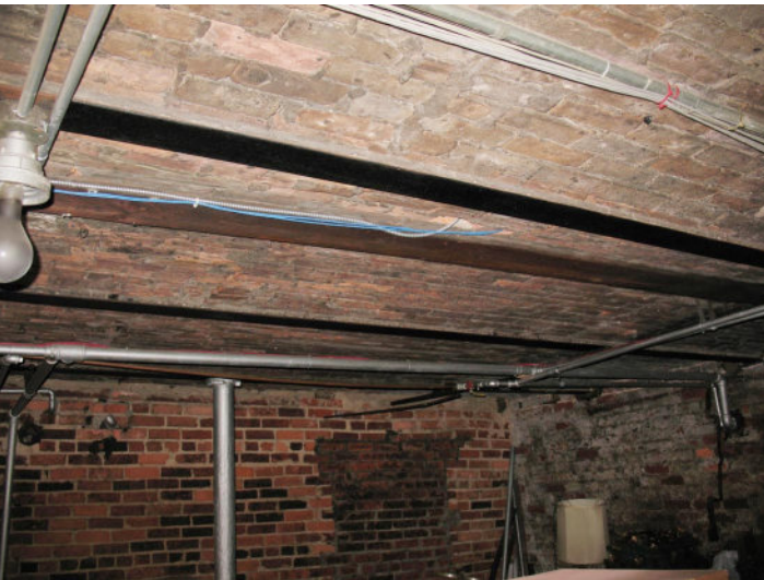
View of first floor brick vault floor structure as seen in the basement.
