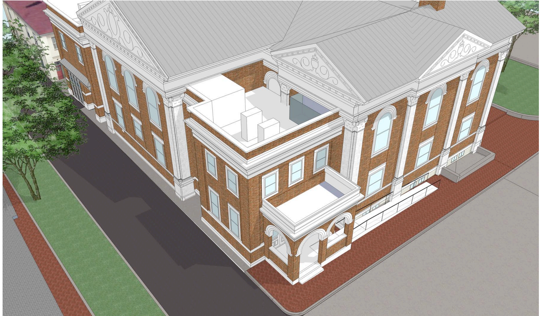
A birds-eye view of the addition on the northwest corner of the courthouse shows how rooftop equipment for the new elevator is screened from view by a parapet wall.
