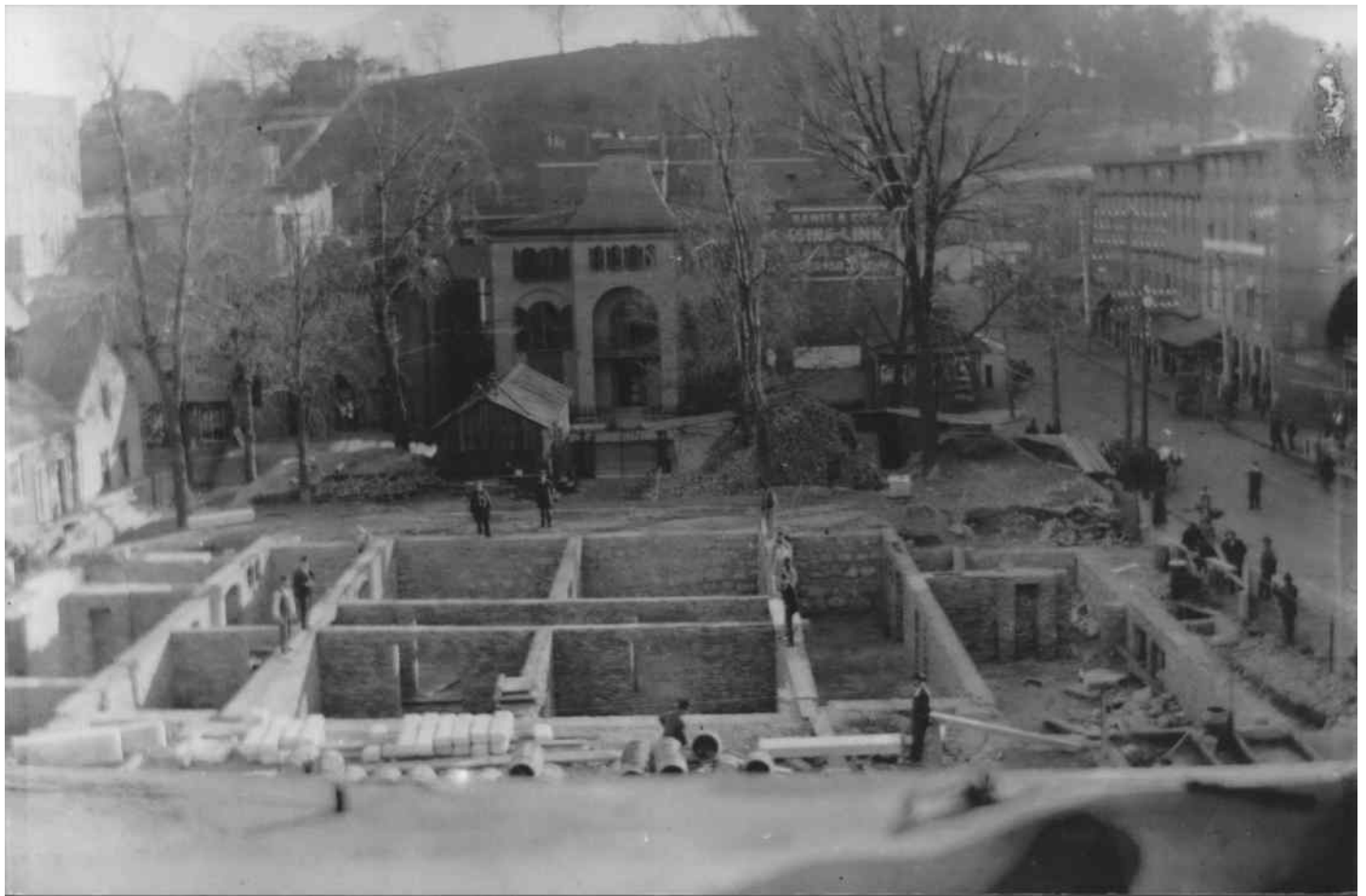
The foundation for the new 1901 courthouse under construction is shown here with the old jail (demolished) across Johnson Street in the background. Hamrick Collection
