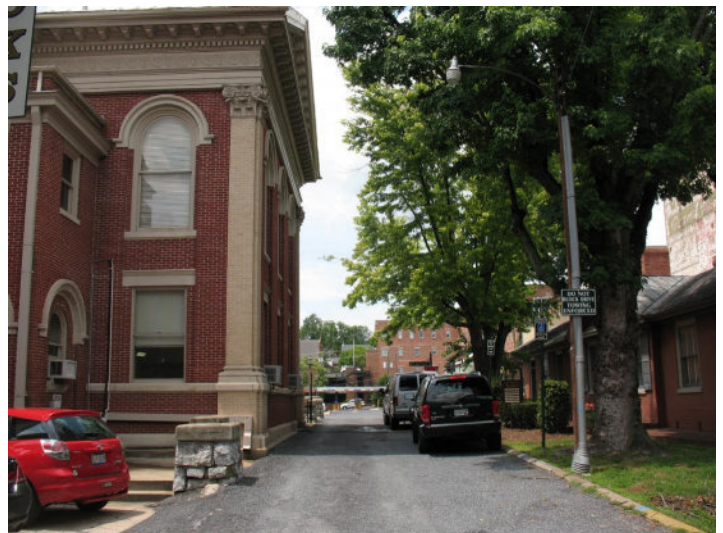
View to the west along Barristers Row alley to the rear of the building.
