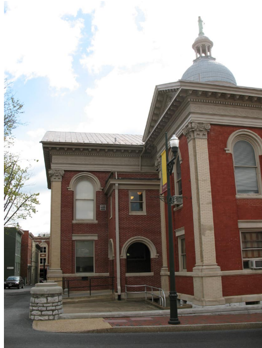
This side view of handicap ramp above shows the incline of the ramp.
