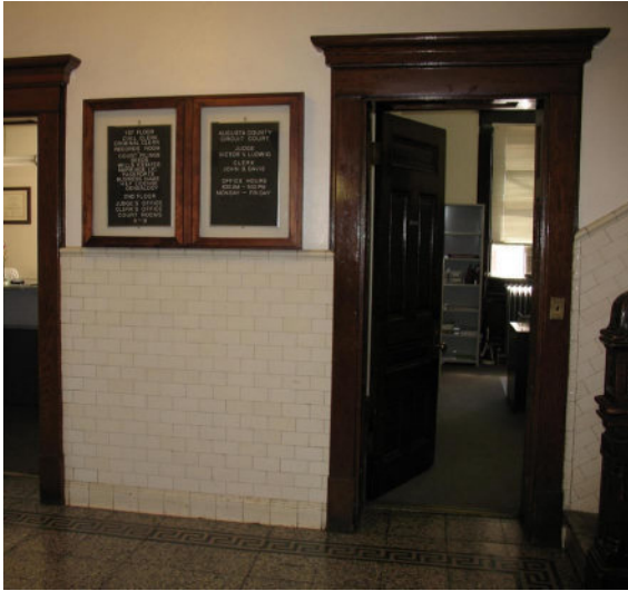
Historic door surround and tile wainscot in the first floor corridor.
