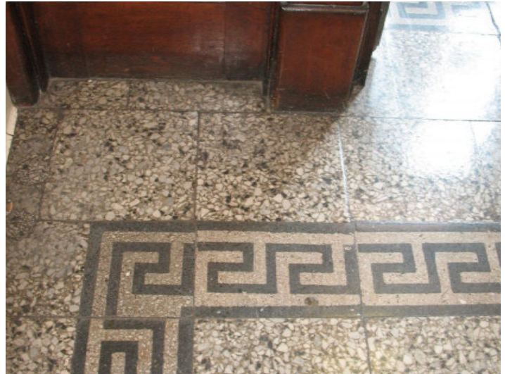
Detail of terrazzo tile finish in first floor corridors.
