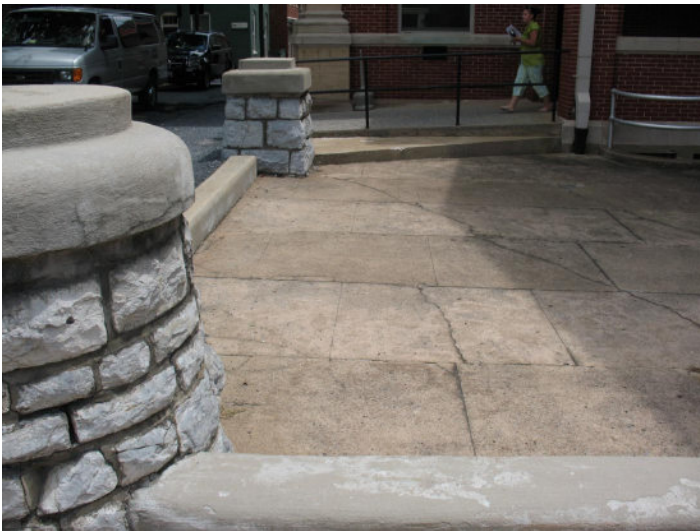
Limestone piers and concrete plaza at the northeast corner of the building.
