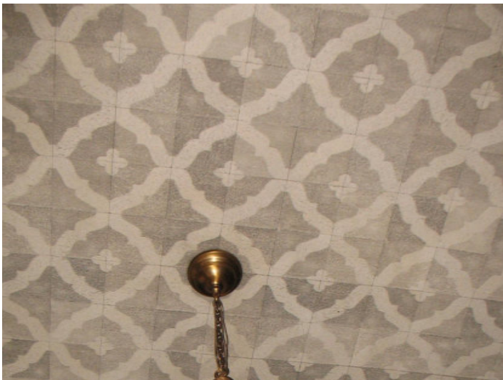
Acoustical ceiling tiles installed during 1949 courtroom renovation.
