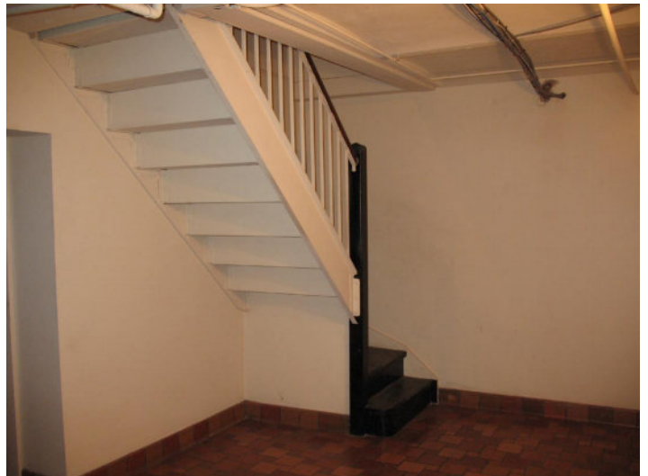
Stair from first floor to basement.
