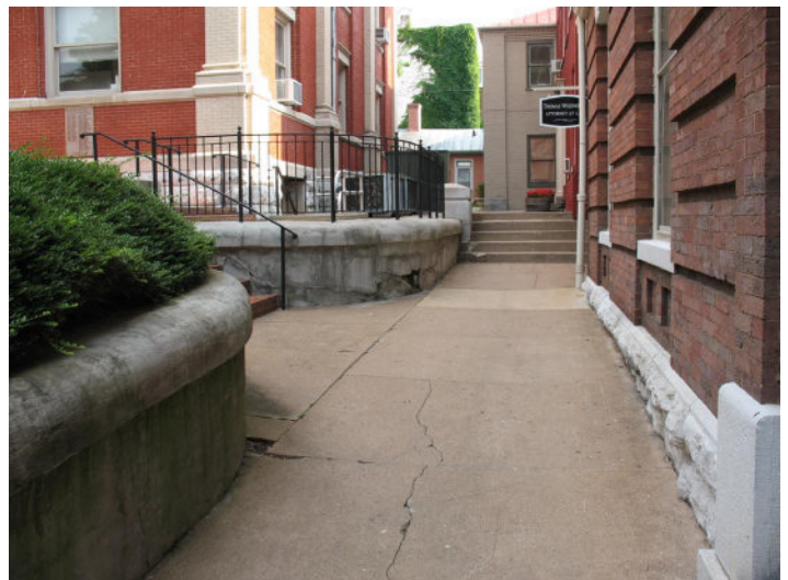
Concrete sidewalk and retaining walls between courthouse and Lawyers Row.
