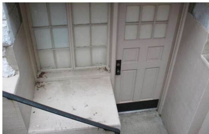
Detail view of exterior stair to basement on the east side of the building.
