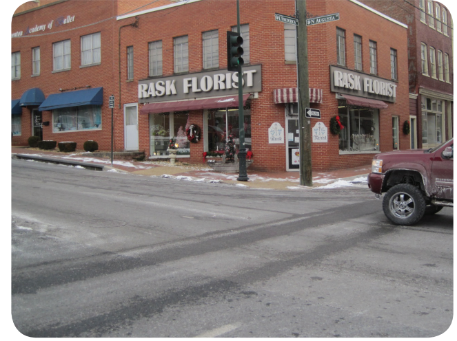
LACK OF ADA COMPLIANCE
