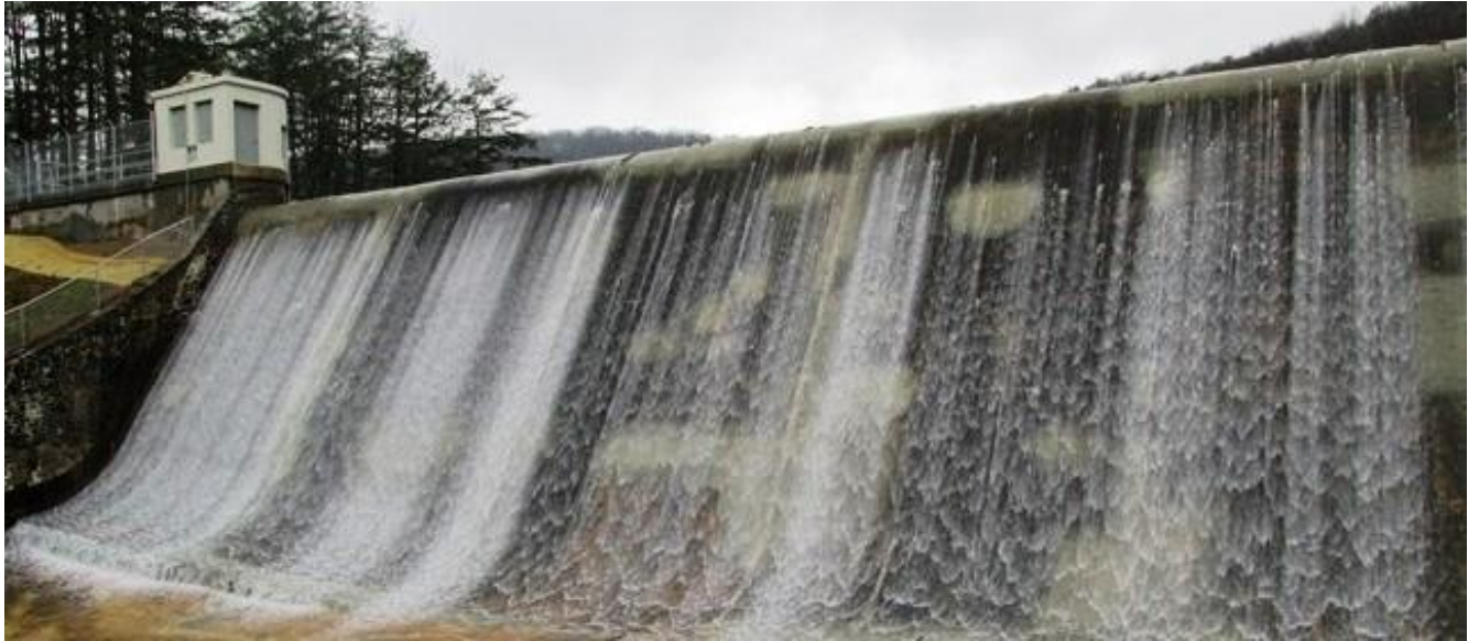
Staunton Dam - One of the City's water sources
