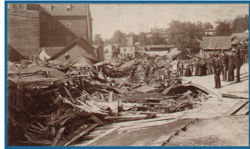
Damages From 1896 Flood (Source: City of Staunton—Local Citizen)
