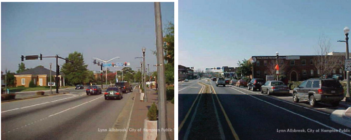
Example of Road Diet, City of Hampton, VA
