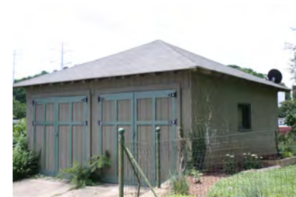
The original wood-frame doors were retained on this historic garage.
