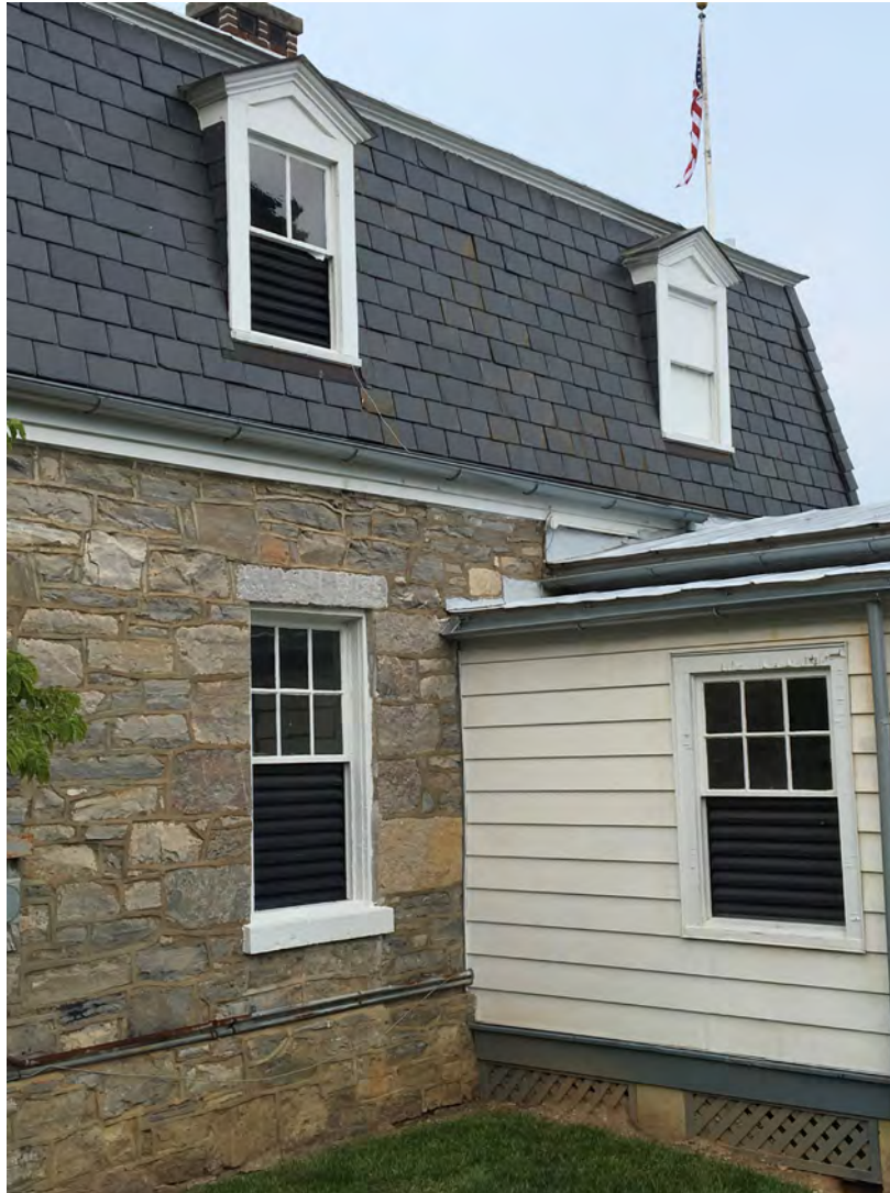
This historic house at the cemetery on Richmond Rd. has been mothballed using vents in the windows to provide air circulation & prevent moisture & mold.
