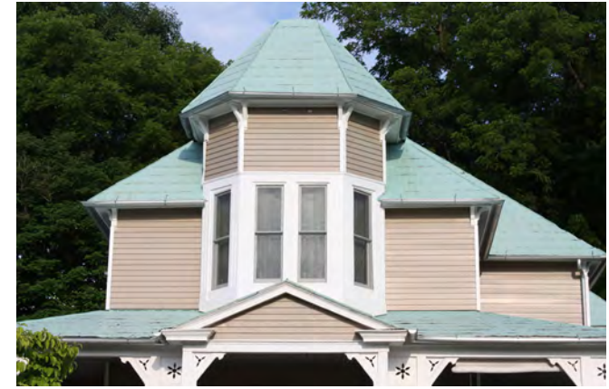
This complex metal shingle roof is a very visible & important element in this historic house's design. It has a central tower, peaked roof, connecting hipped roofs, & a hipped porch roof with a gable roof over the entry.
