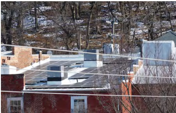
Solar panels, recently installed on this Wharf building, are not very visible and have limited impact on historic fabric.
