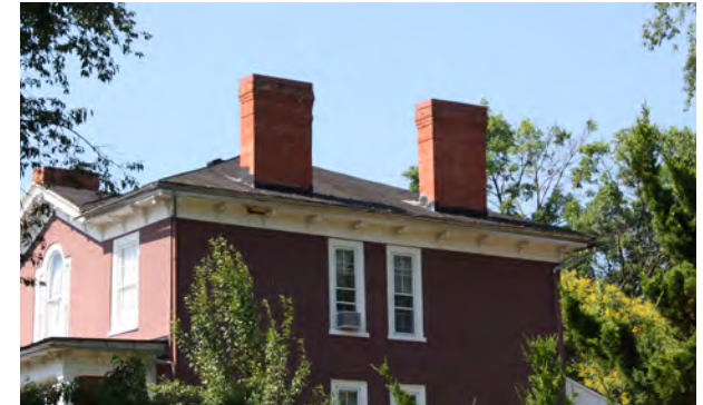
Double interior end chimneys.
