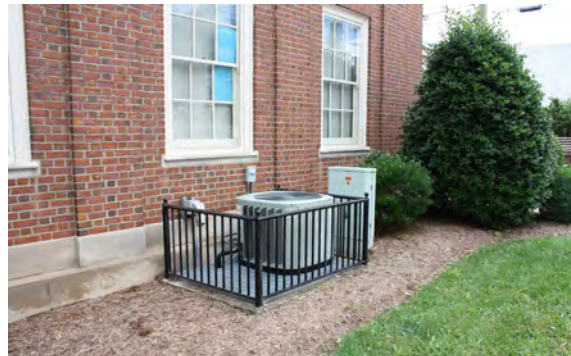
This HVAC compressor is protected by a painted metal fence but not screened because of air circulation requirements.
