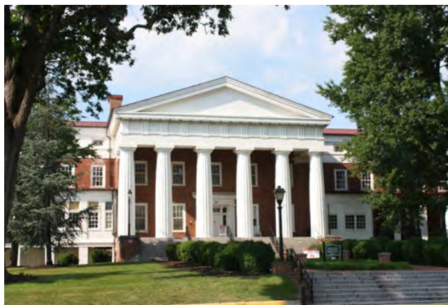
Staunton's most prominent example of a Greek Revival building with its Doric portico is the Virginia School for the Deaf & Blind (VSDB). It is also one of Virginia's most important examples and was completed in 1846. VSDB was designed by the Baltimore architect, Robert Cary Long.
