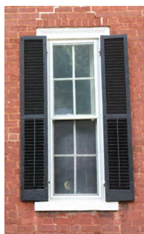
Four-over-four sash in a late 19th c. brick building.
