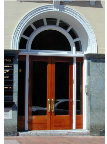
Double commercial door with sidelights & semi-circular arched transom.
