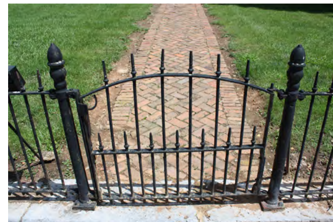
Cast iron gates with decorative features help define the entrance to many residences in the historic districts.
