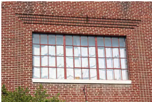
Steel frame casement windows arranged in a set of three 16-light windows with a center four-paned section that opens for ventilation.
