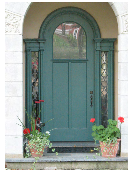
Leaded glass patterns on these sidelights are an important decorative detail to this entrance.
