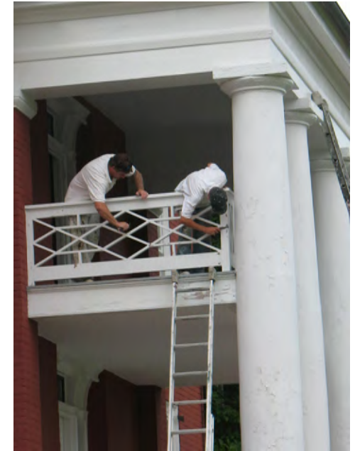
This trellis porch railing is being prepared for painting to ensure long-lasting protection of the wood.
