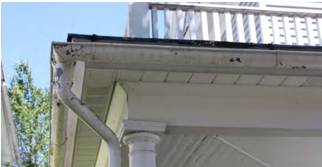
Galvanized gutters & downspouts must have the proper primer, or the paint coat will not adhere to the metal.
