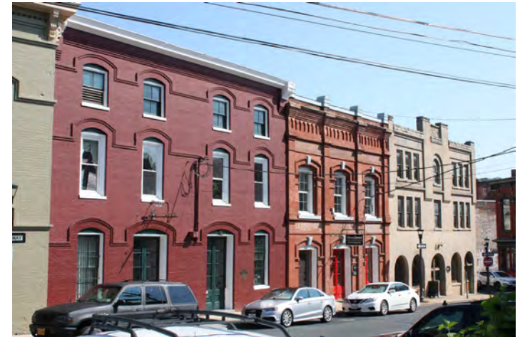
Wharf Area Historic District warehouses create a street wall and have a variety of brick details.
