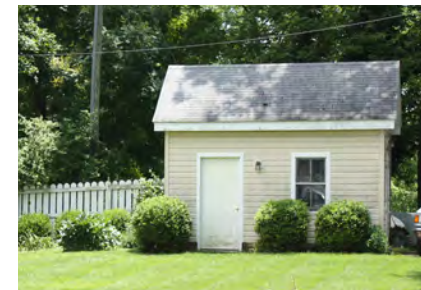
A typical and appropriate garden shed with simple frame construction & a gable roof.
