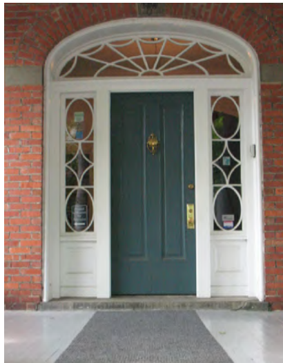
Two vertical paneled door on this Colonial Revival styled house.
