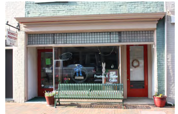
This storefront retains its prism glass tile transom, a rarely surviving feature. Note the door to the upstairs space.
