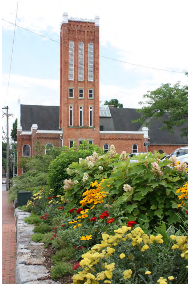
Parking lots in the historic districts are well maintained & this example has attractive seasonal plantings.
