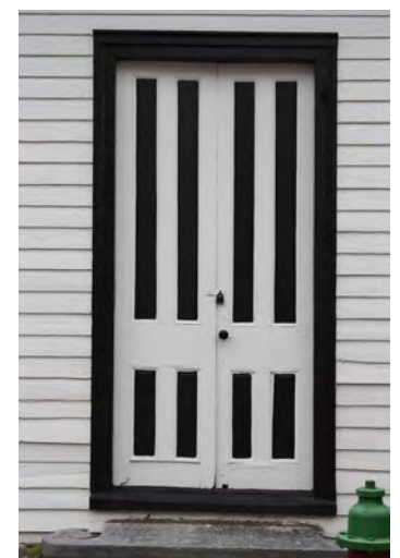
Typical Victorian era warehouse doors with a set of four-paneled doors.
