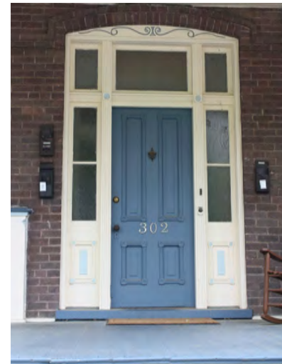
Typical Victorian era entry complex with a four-paneled door flanked by paneled sidelights & a divided transom formed by the framing.
