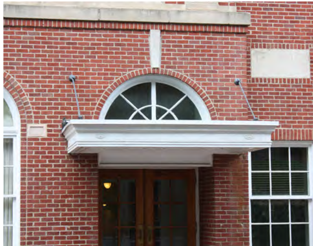
This small canopy is supported by metal cables & provides protection over the primary entrance to this hotel.
