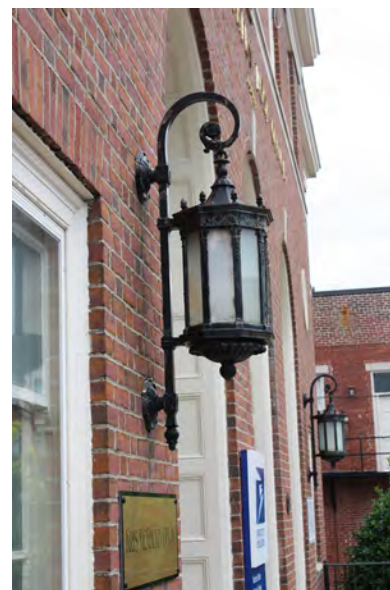
This pair of ornate cast-metal light fixtures are important character-defining elements to this property.
