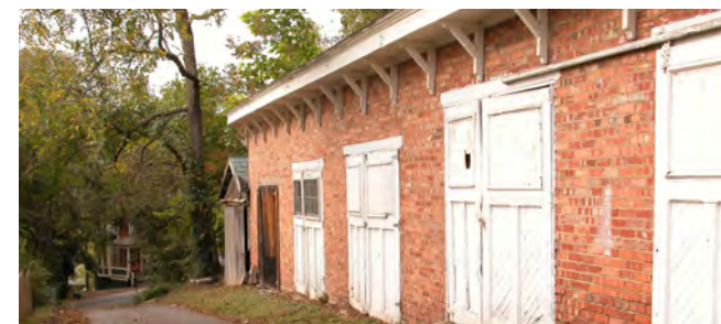
This brick garage with multiple vehicle bays has a shed roof with an overhang supported by decorative brackets. There are several other larger garage complexes in the historic districts like this example and they are a unique historic outbuilding form.
