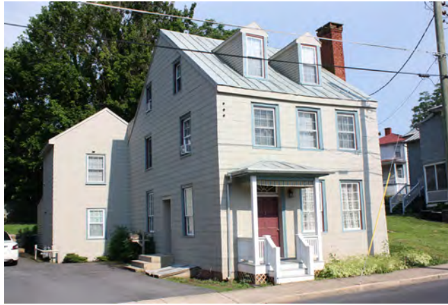
This N. Augusta St. dwelling is a Federal styled rowhouse & is constructed of logs, later covered with asbestos shingles.
