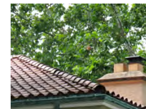
This is a rare example of a clay tile roof found in Staunton's districts.
