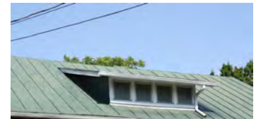
Shed roof dormers often are a trademark feature of the bungalow style.
