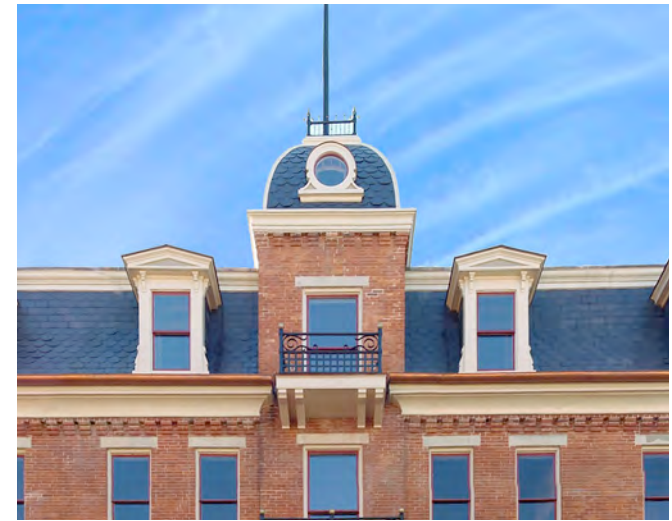
Artificial slate was used as a replacement material on the roof of the R. R. Smith Center for History & Art. This substitute material is recommended only when the existing slate has deteriorated beyond retention. The artificial product is to be used on taller structures where the detail & texture of real slate cannot be perceived from the ground level.
