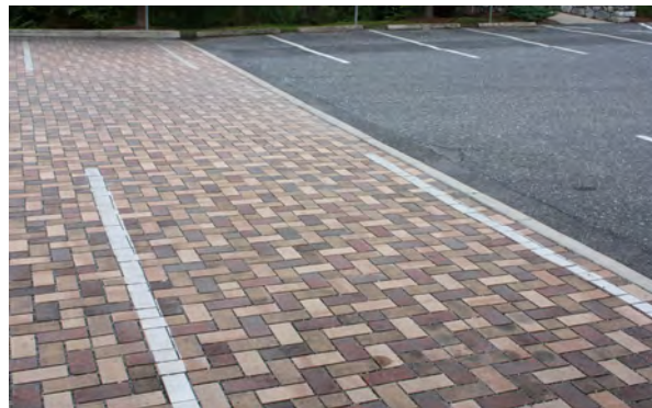
Permeable pavers are used with contrasting bricks to divide the spaces in this parking lot. This design helps reduce water runoff & the pavers are a more appropriate material than the asphalt paving.
