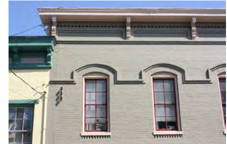
Raised brick belt coursing continues around the segmentally arched windows of this warehouse.
