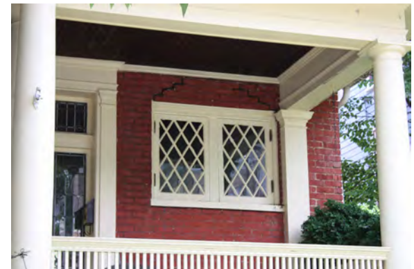
This pair of small casement windows contains decorative diamond shaped panes.
