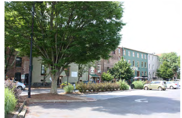
The north (rear) elevations of these Wharf warehouses have additional lower levels due to the grade changes from Byers St. to Middlebrook Ave.
