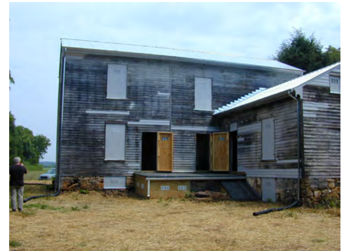
The mothballing of this historic house included enclosing openings with plywood for security purposes. The windows' plywood panels included vents to allow for ventilation.
