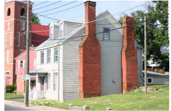
A pair of exterior end chimneys.
