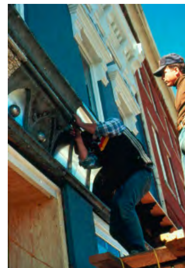
Deteriorated parts of a metal cornice are being carefully replaced.
