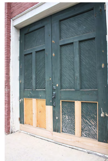
Only deteriorated parts of an element should be repaired or replaced, not the entire doors.
