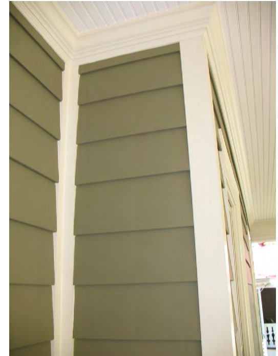
Contemporary products that replicate historic materials have become more popular & include items like this fiber cement siding example.
