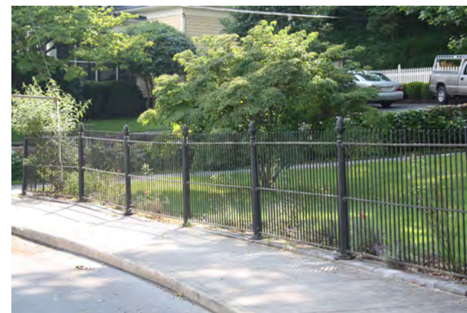
This historic cast iron metal fence with acorn finials on the posts provides another unique feature to this site.
