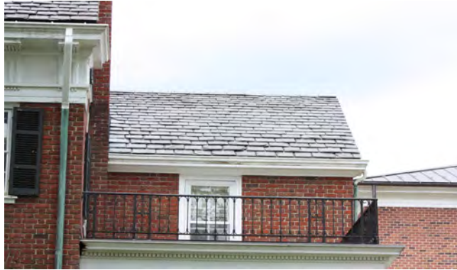
This roof is clad in a typical pattern of Buckingham slates that have a life expectancy of approximately 150 years.
