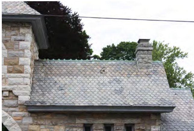
This roof has a shingle pattern of Pennsylvania slates, & their life expectancy usually is less than 100 years.
