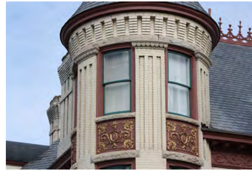
Corbelled brickwork, recessed brick panels, decorative panels, & roof cresting are just some of the details of this ornate residence.
