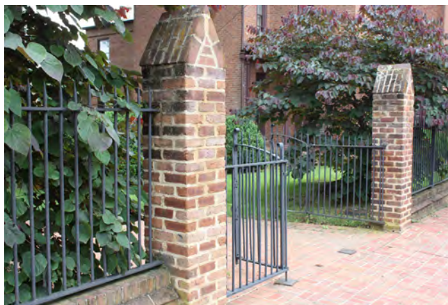
This low brick wall, brick piers, and a metal fence are important historic elements defining this church yard.
