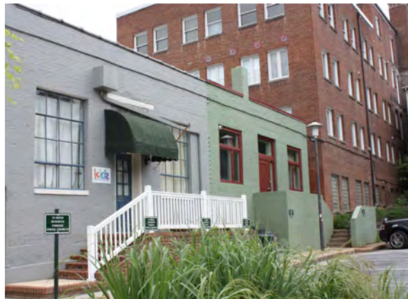
These rear additions were redesigned to create two new rental spaces for separate tenants. They become new facades for the businesses within them.
