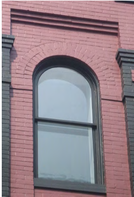
Windows & doors are recessed in masonry openings as seen in this arched example.
