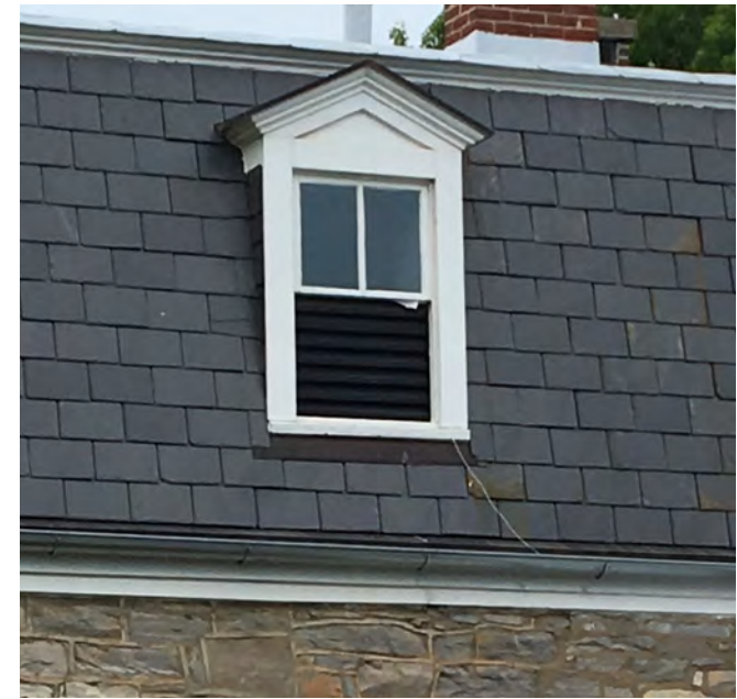
Window ventilation is an important element to install in a mothballed historic building.
