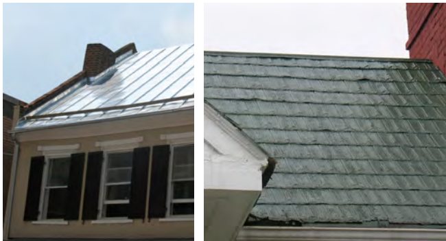
Standing-seam metal roofs are very frequently used in Staunton's historic districts (left) while metal shingle roofs (right) are less common.
