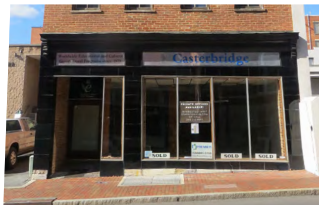
Structural pigmented glass panels used on this late 19th c. building's storefront was an early 20th c. upgrade during a remodeling.
