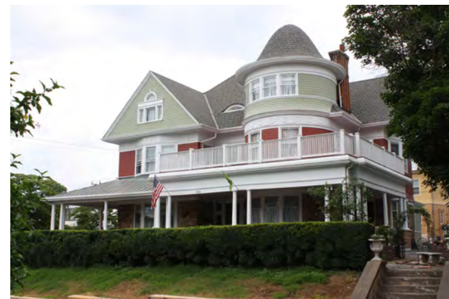
This Queen Anne example has a more unified design with a classically designed wrap-around porch & shingle clad surfaces. The decorative cornice has classical motifs as well. With these features, the design might also be classified as one of Staunton's rare examples of the Shingle style.
