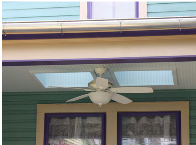
This fan light helps to illuminate an outside porch while providing ventilation for this residence.
