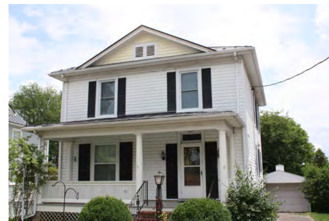
This American Foursquare frame house has a wide roof gable instead of the typical dormer found on most examples of this style.
