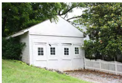
This wood framed garage still has its unusual doors with small paned windows.
