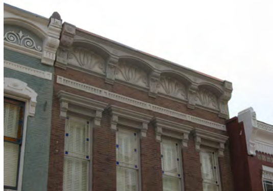
Painted, galvanized metal, decorative details like this floral patterned, bracketed cornice & window caps are present on many of Staunton's commercial buildings.
