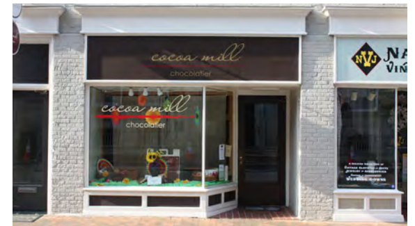
Likely, the interior of these storefronts has a lowered ceiling and therefore the transom became an appropriate location for signage.
