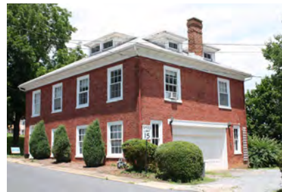
Another example of a studio use on the upper level of this brick carriage house.
