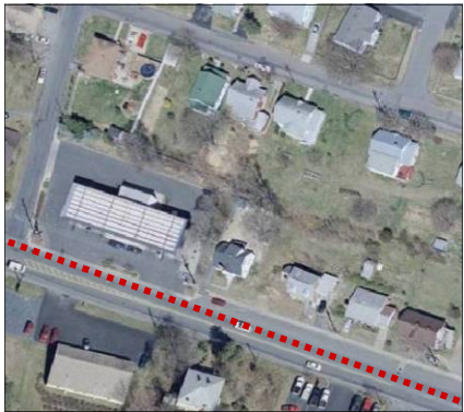
houses and neighborhood corner gas station share coordinated setbacks
