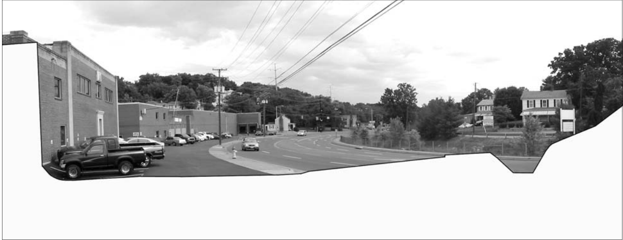
Section e: existing conditions
