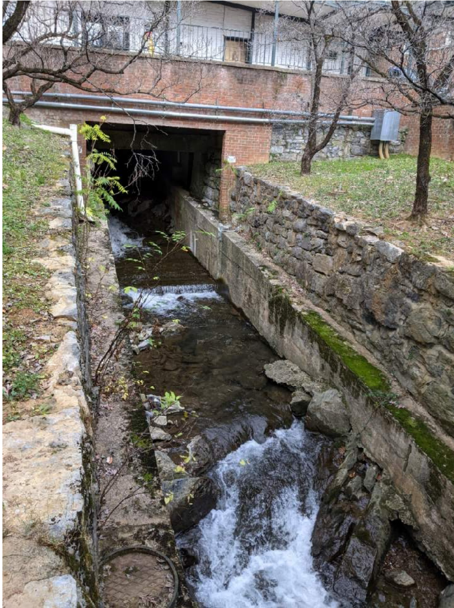
Photo 11 – Creek opening between garage and City Hall, looking upstream
