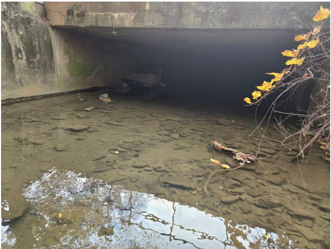
Photo 6 – Byers St, at culvert opening
