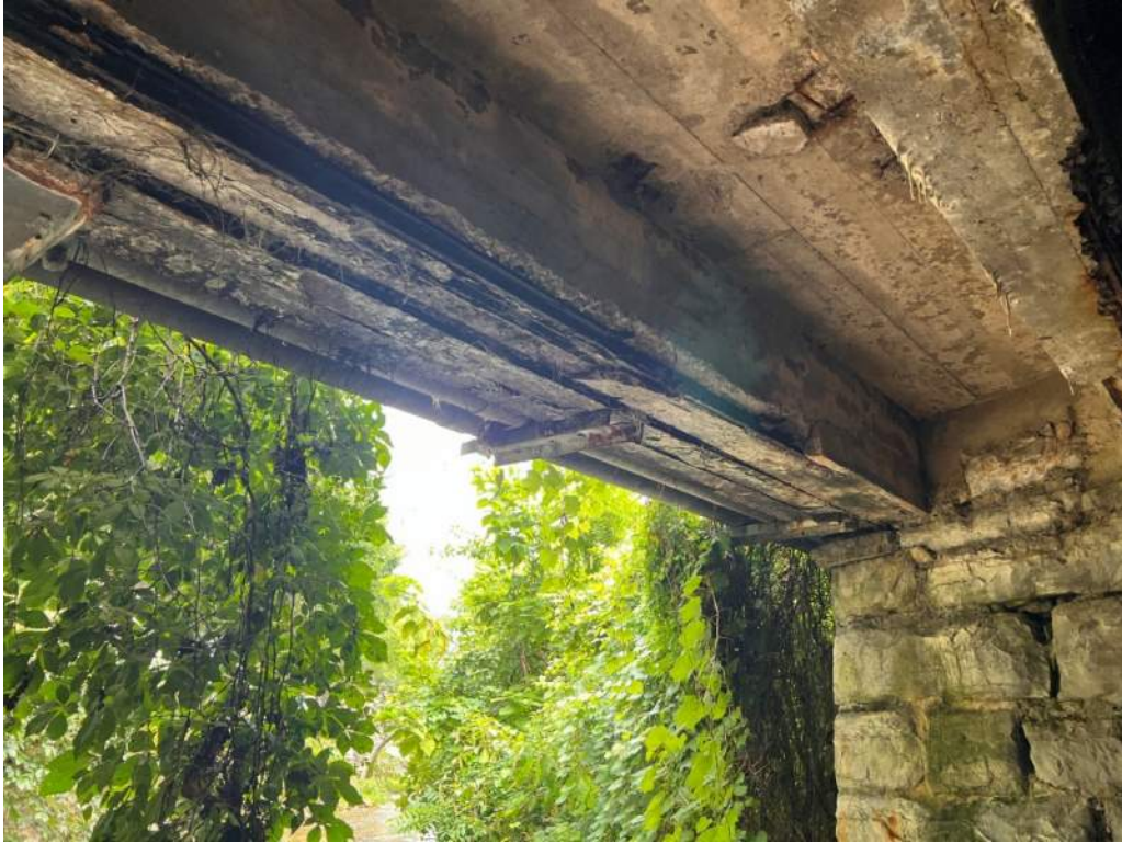
Photo 9 – New Street, near end of tunnel, looking south
