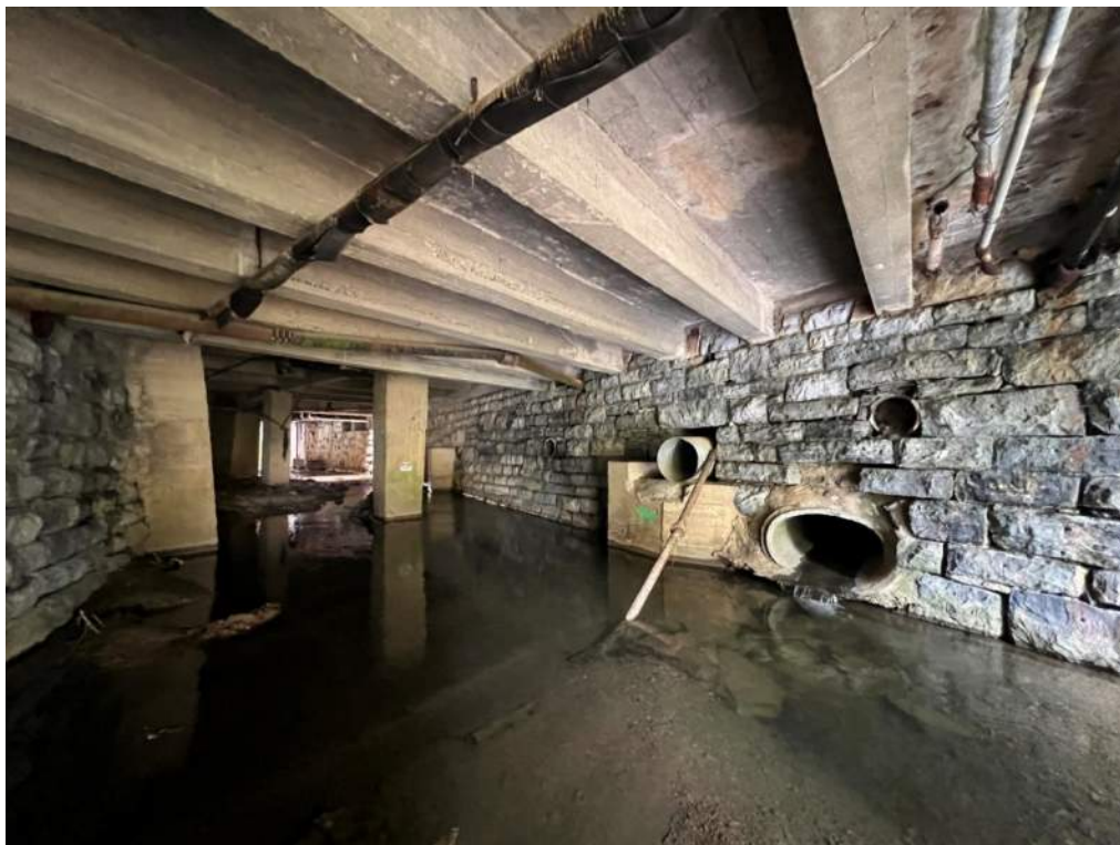
Photo 8 – New Street, near end of tunnel, looking upstream
