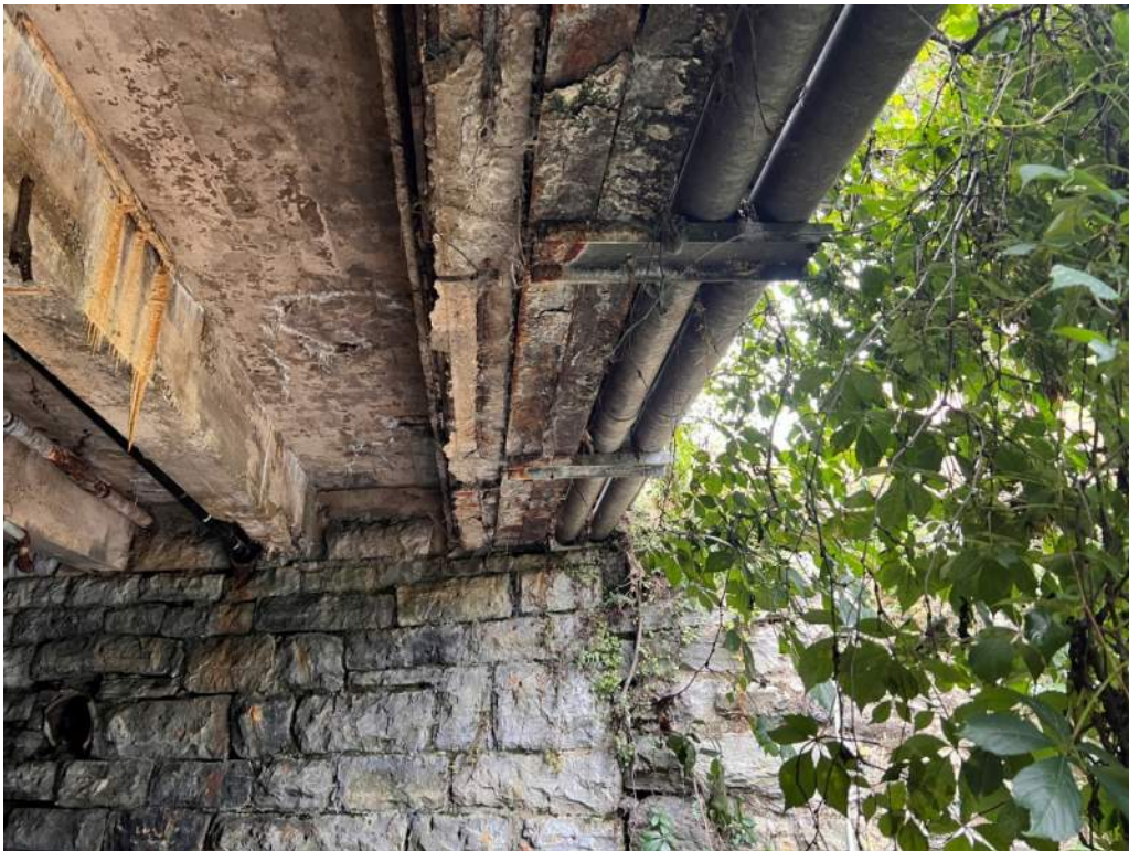
Photo 10 - New Street, near end of tunnel, looking north
