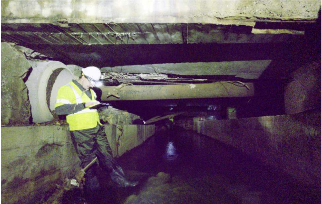
Photo 1 – Johnson Street at Garage Entrance looking Downstream
