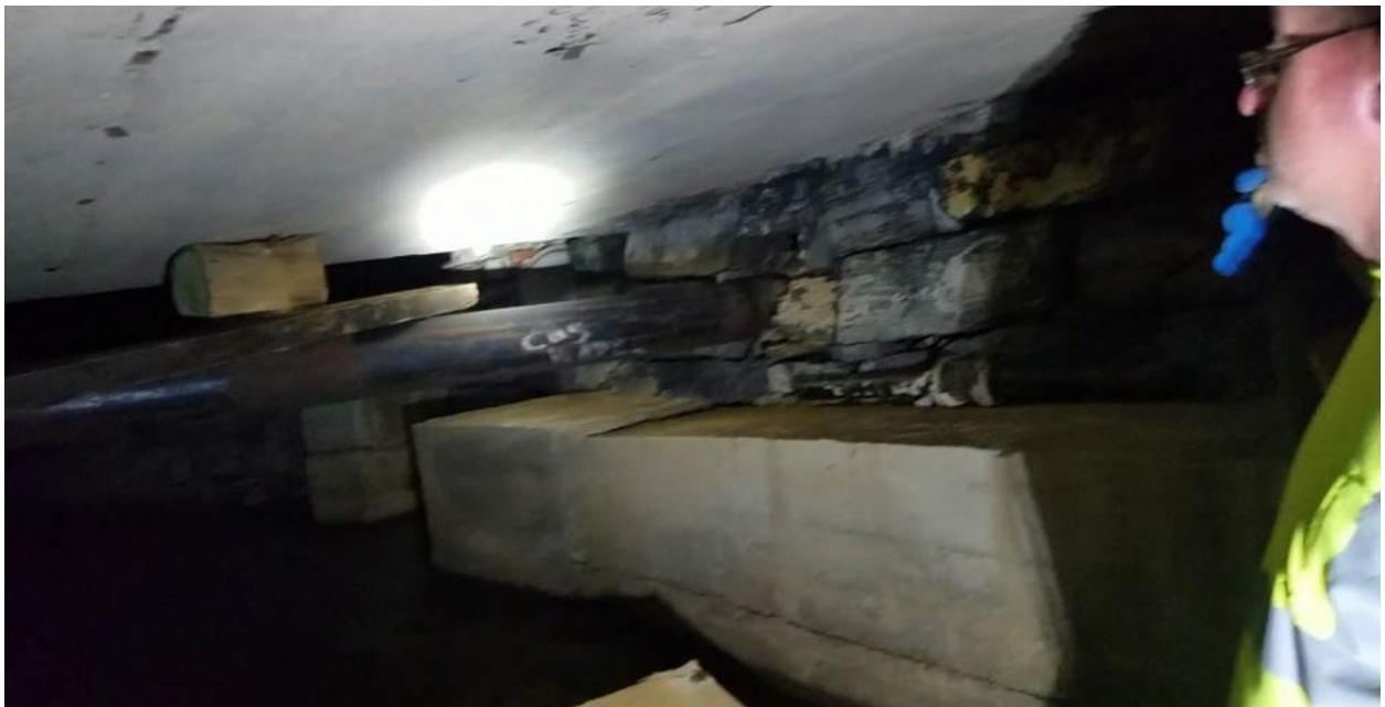
Photo 4 – Johnson Street, Water line and sewer, looking downstream
