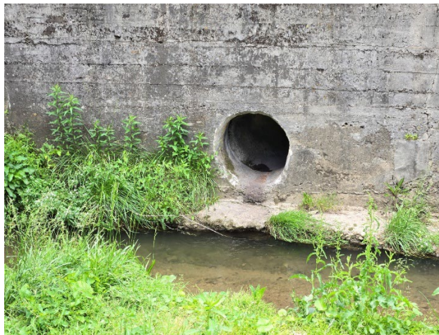
Photo of outfall taken during IDDE inspections.
