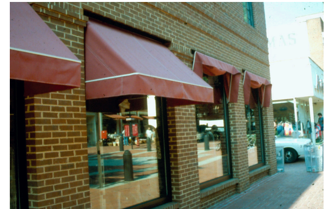
Fabric awnings can be fully retractable or pulled back such as this example.
