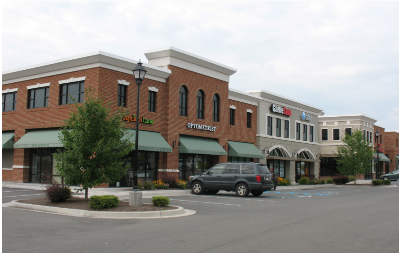
The varied-height roof lines in the new development above conceal sloped roofs that are surrounded by decorative parapet walls.
