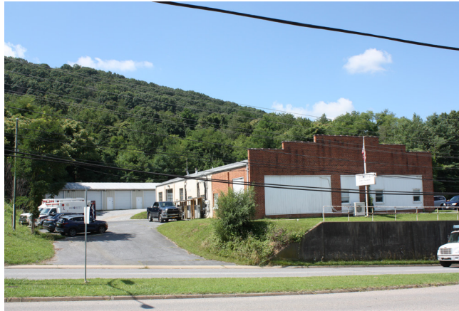
The older structures on the south side of Richmond Avenue west of Bell Street are sited on raised parcels, typical of this portion of the corridor.
