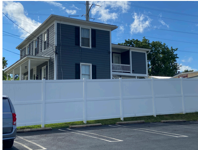
Above: This example of a high-quality wood fence separates the parking area of a commercial corridor building site that adjoins adjacent residences.
