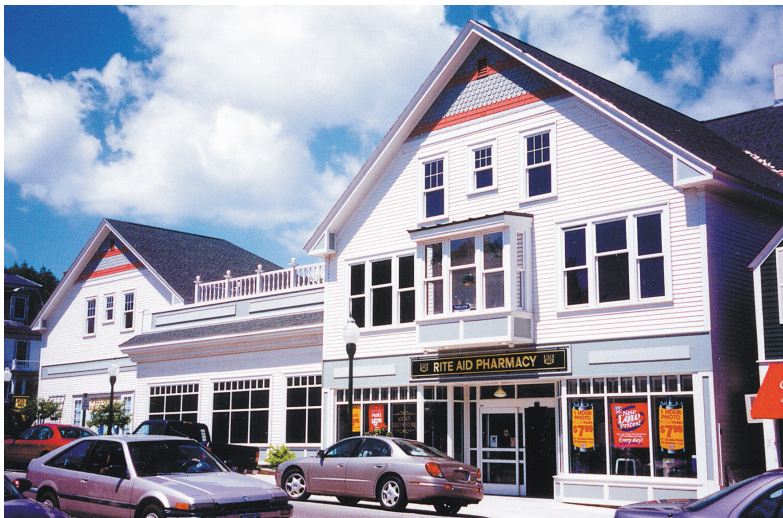
This gable roof option is a more traditional design treatment for a newly constructed national pharmacy chain building.
