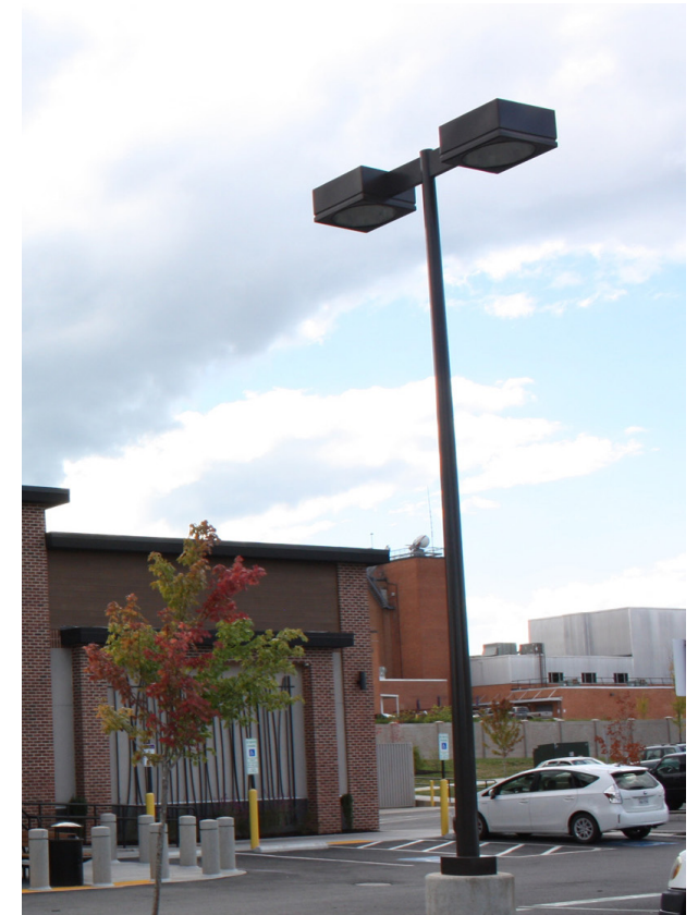
This parking lot uses taller shielded fixtures to illuminate larger sections of the site.
