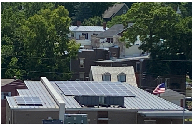
This local example on N. Augusta Street shows the slope of the solar arrays to be the same as the roof slope (left) making the arrays not visible from the street level as shown in the photo at right.
