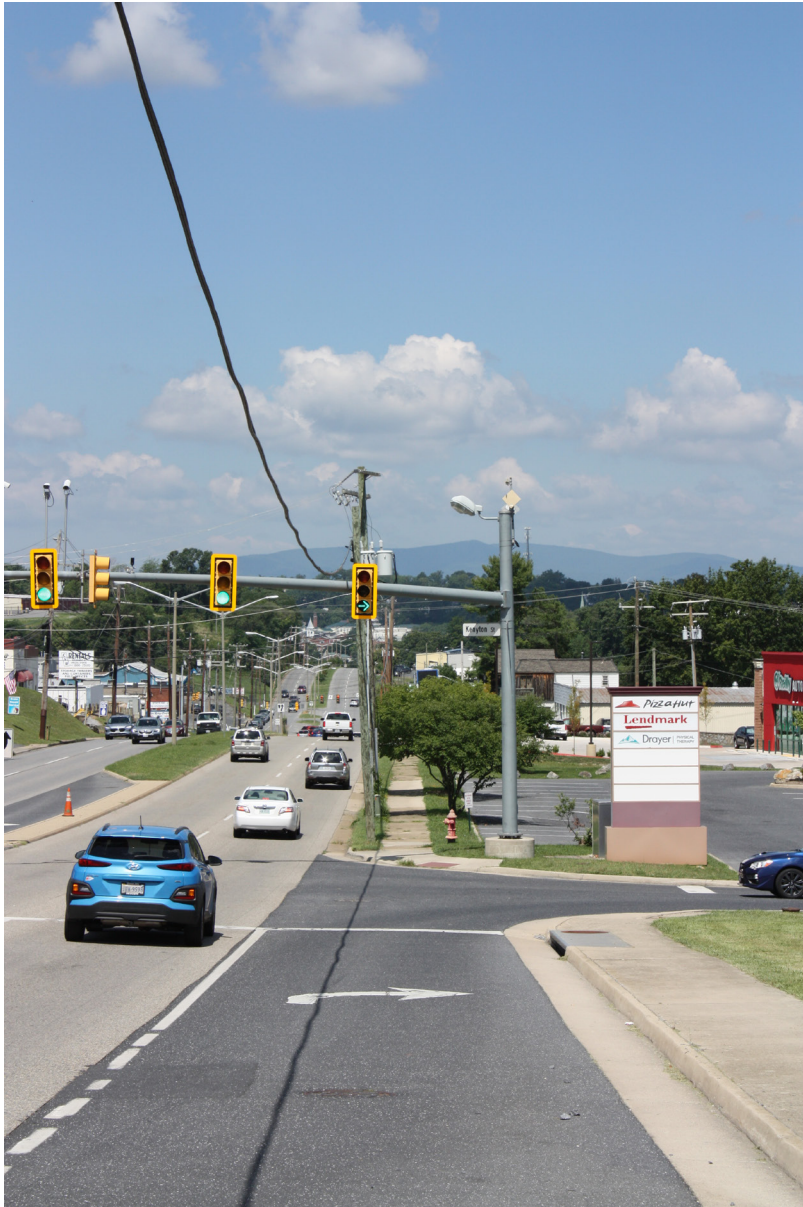
Richmond Avenue is the most traveled commercial corridor in the city and as a result, has seen the most new development of all corridors.
