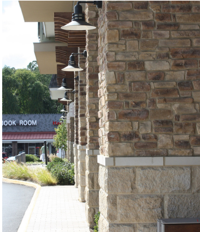
These shielded lighting fixtures on a facade light, not only the stone piers, but also the pedestrian path along the building. This parking lot uses taller shielded fixtures to illuminate larger sections of the site.
