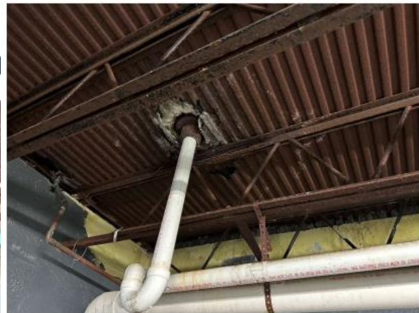
Figure 10 Delaminated Open-Web Steel Joist
