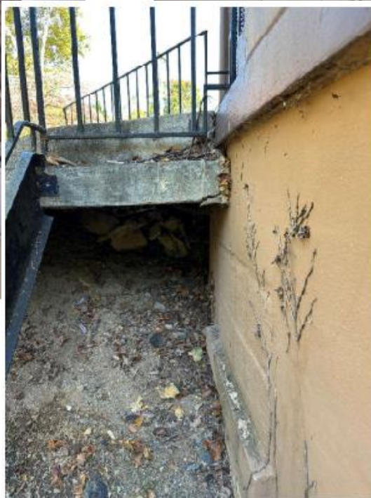
Figure 8 Staff stair landing
