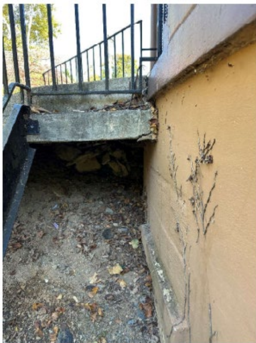
Figure 8 Staff stair landing
