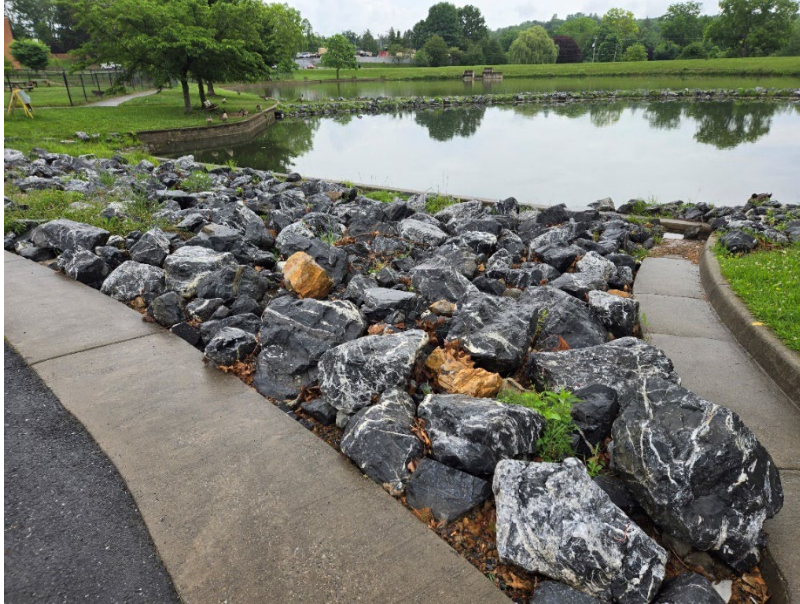
City maintained BMP – “Lake Tams”
