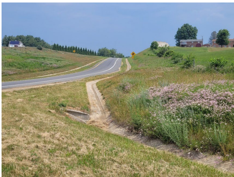
Photo of stormwater conveyance channel taken during IDDE inspections.
