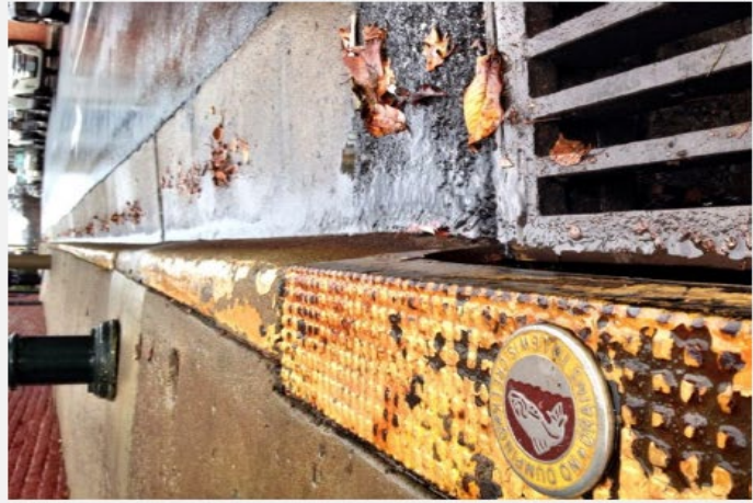
Storm drain in downtown Staunton
