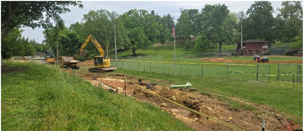
The Gypsy Hill Park Stream Restoration Project is now underway and is expected to be completed in March 2025. This project will help to improve the health of the stream by repairing the damaged channel, stabilizing the stream banks, and planting native vegetation to provide a better habitat for aquatic life. It will also involve measures to slow down the flow of water during heavy rains, which will help reduce the risk of flooding downstream.
