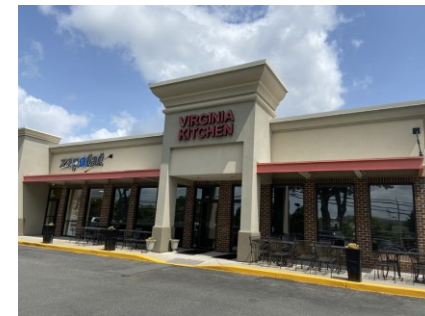
Wall signs for buildings along a corridor are generally well placed on the façade above the storefront so they are visible from passing vehicular traffic.
