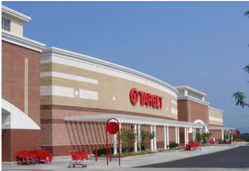
This big box franchise uses various techniques to reduce the scale of the long facade including different size and shapes of the four bays, separate cornice designs, several shades of red and tan for the masonry as well as a pergola protruding from the central bay.
