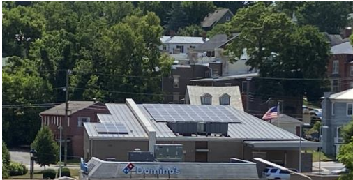
This local example on Augusta shows the slope of the solar arrays to be the same as the roof slope (above) making the arrays not visible from the street level (left)
