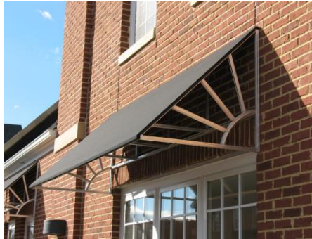
This awnings has a traditional fabric canopy with a contemporary decorative metal frame.
