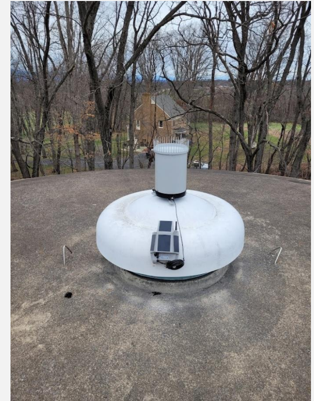
Van Fossen Water Tower
