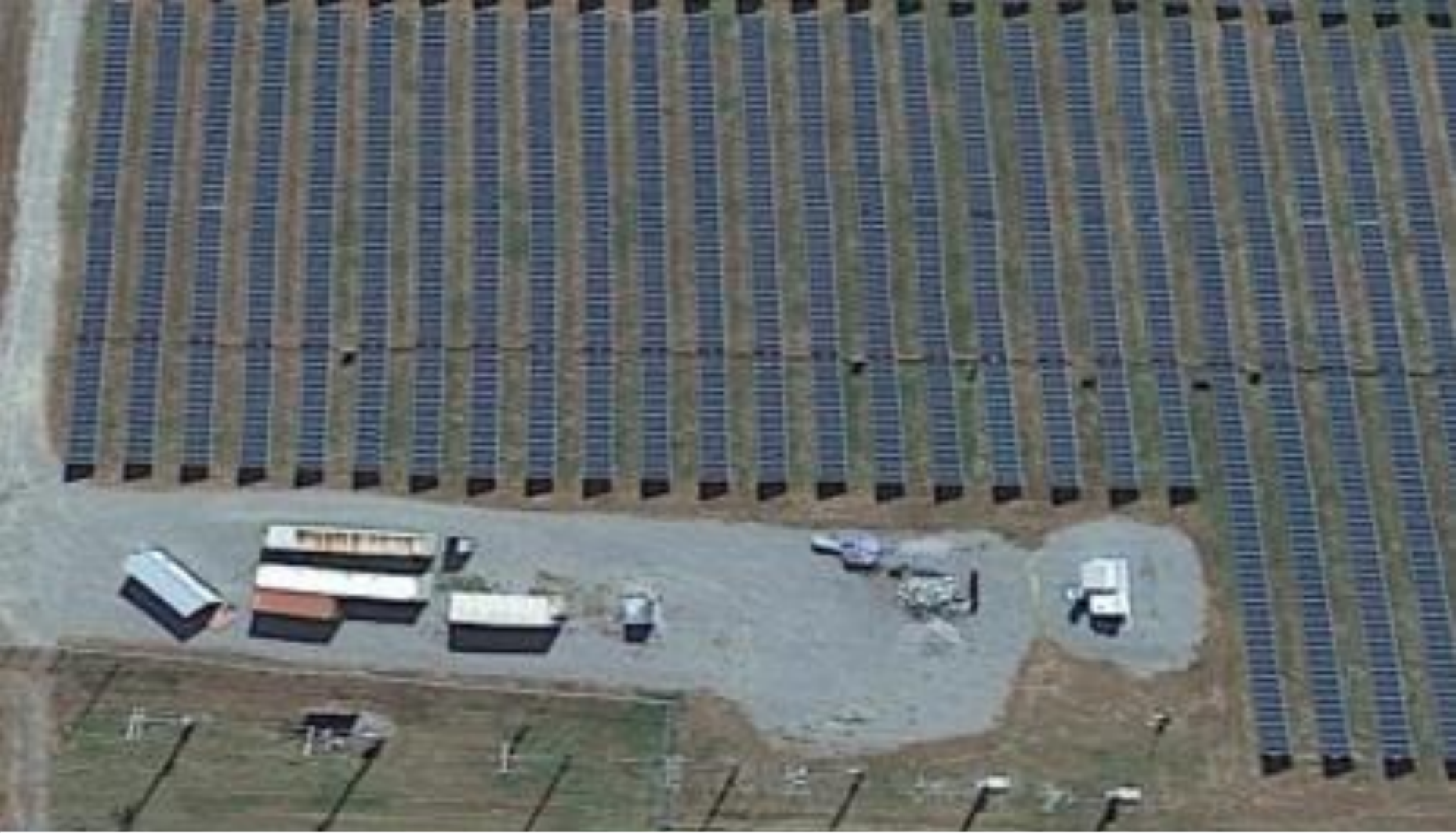
Collection Station for 20 MW Solar Facility in Stony Creek, VA
