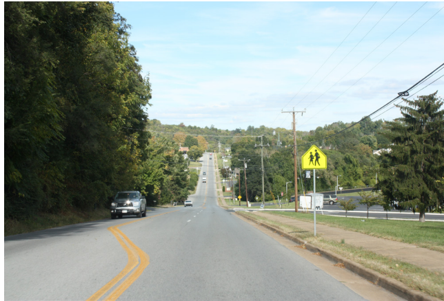
This view is looking south on Coalter Street showing side-walks and mature landscape.
