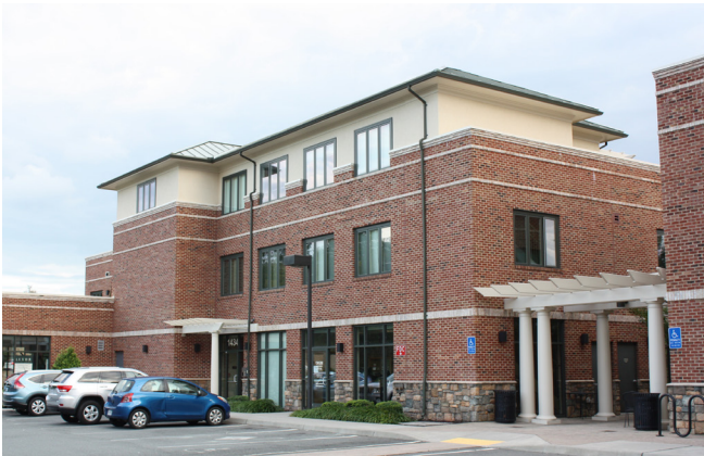
This example accentuates the foundation with stone creating a visual base for the brick building.
