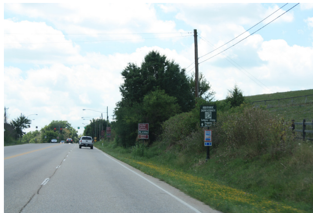
Another view looking south showing the rural setting and customized welcome and directional signs which are located on most of the city's corridors to welcome and direct visitors.
