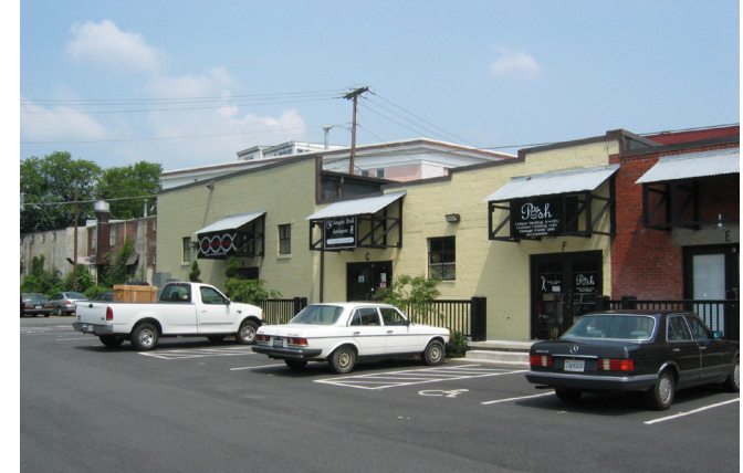
These contemporary canopies provide identification of different business entrances as well as a place for signage.
