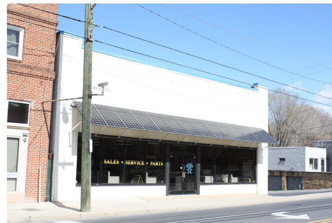
Solar panels can also be creatively used as storefront awnings as shown in this second local example.
