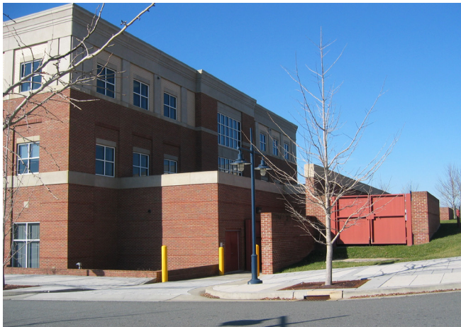
Mechanical equipment at ground level and visible from the public right of way should be screened such as this example.
