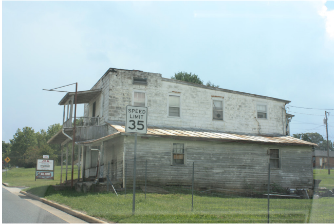
At the entrance to Staunton on Churchville Avenue is an example of an early commercial building.
