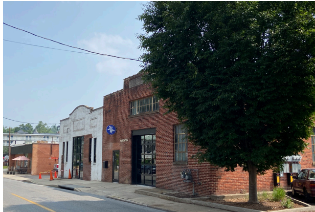
This view looking north on Lewis Street shows early warehouse buildings, many of which recently have been renovated and contain new uses.
