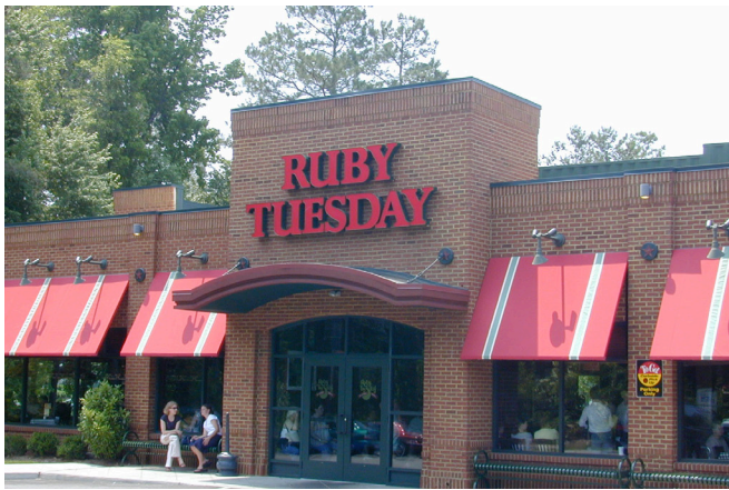
This is an example of a standard sloped fabric awning that gives the business a colorful accent.
