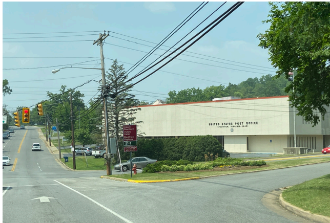
The U. S. Post Office is located on Augusta Street at the intersection of Lambert Street. Surrounding uses include residential and commercial.
