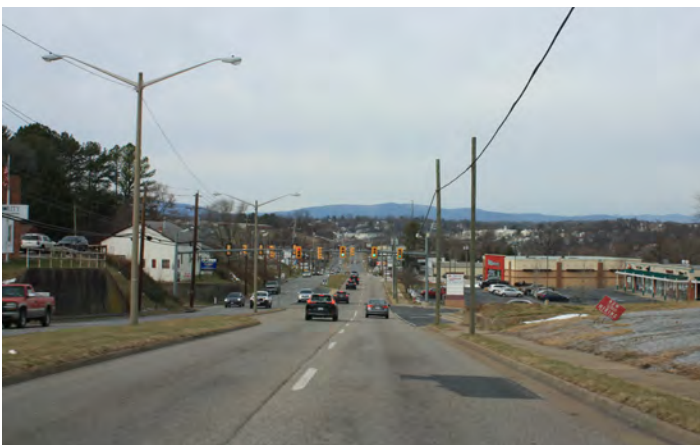
Further west on the corridor, a planted median divides the four lanes and a sidewalk has been installed on the north side.
