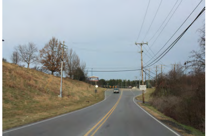
The steep slope of the west side of the corridor still contains a motel and further north access to the Lowe's retail establishment.
