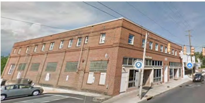
This two-story mixed use building (now Valley Mission) on West Beverley Street with its storefronts is a historic facade design.
