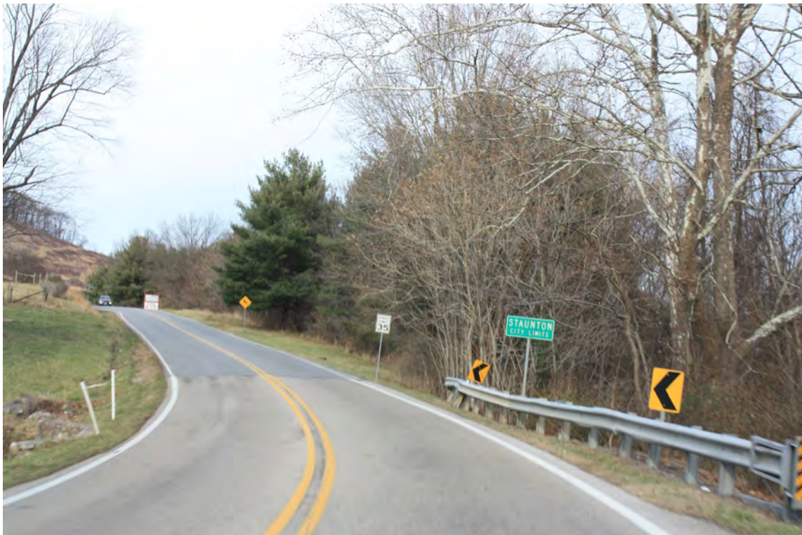
Frontier Drive remains rural along much of its route due to steep slopes and the western boundary of the American Frontier Culture Museum parcel.
