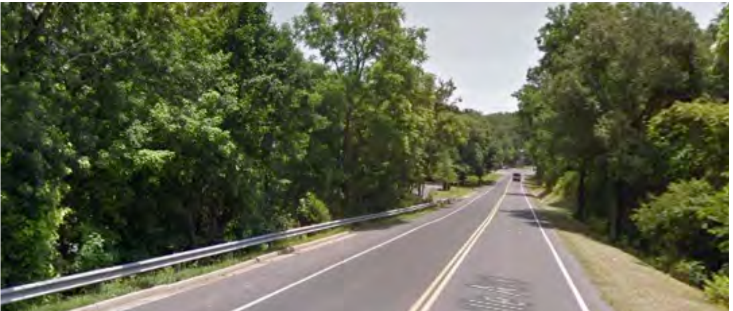
Headed west, Churchville Avenue becomes a rural highway at the City limits.
