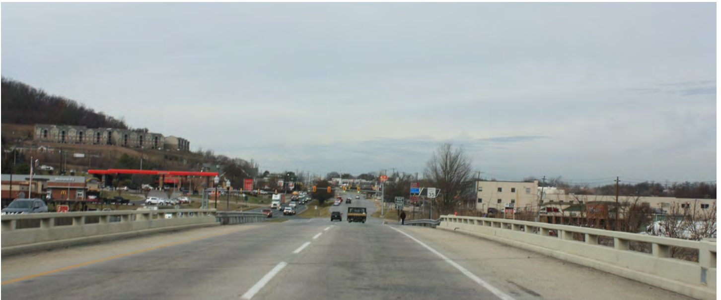
Richmond Avenue is a major entry route to the city but lacks any significant gateway welcoming features. The city-owned Betsy Bell Mountain recently has become encircled with a large multi-family complex. A mixture of recent fast food franchises, gas stations and other retail line both sides of this growing commercial corridor.
