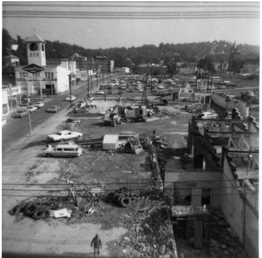
The Central Avenue corridor (looking north in this photograph) experienced radical changes in the 1960's when all of the businesses and residences on the east side were demolished for an urban renewal project which remained vacant for years.
