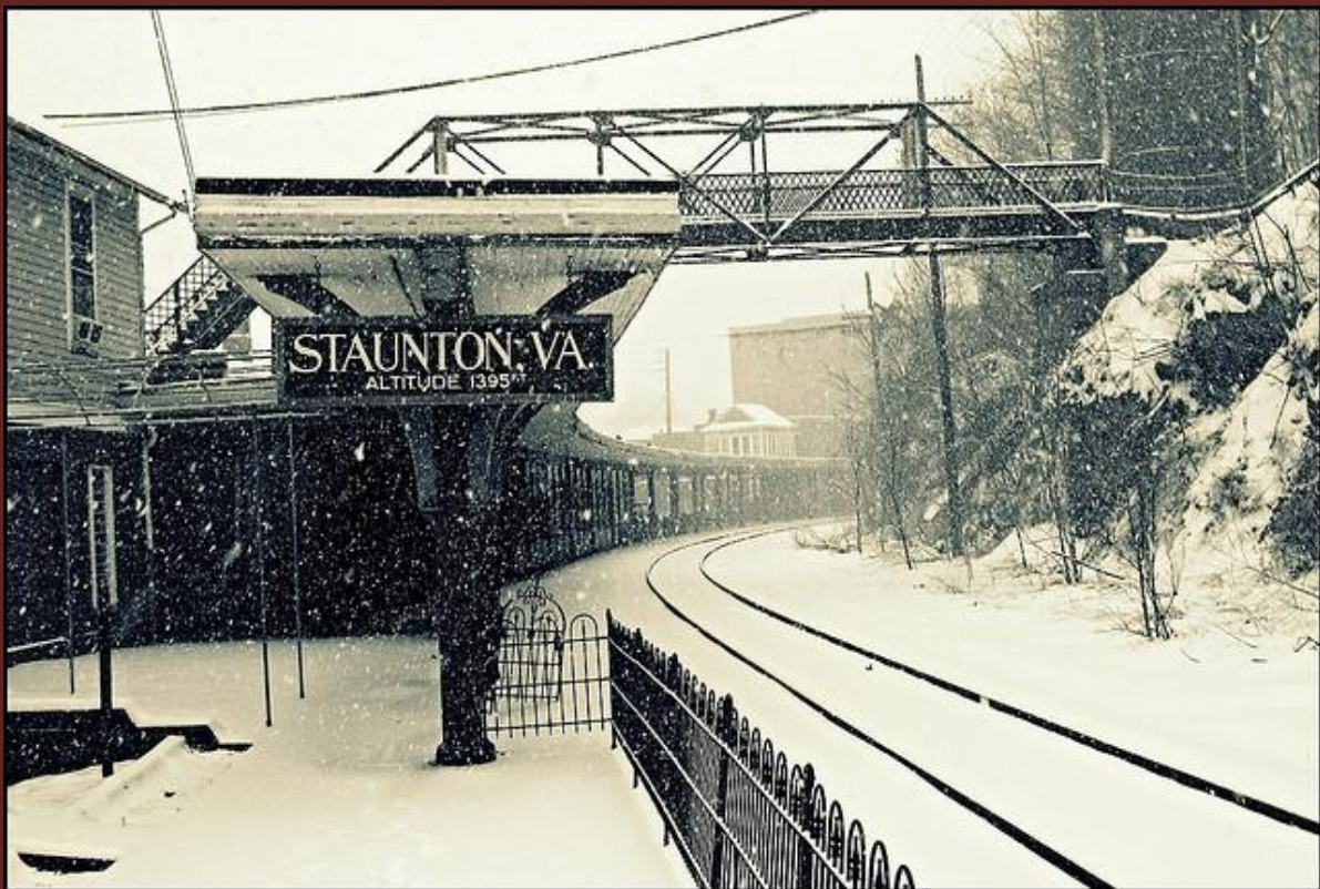
Sears Hill Bridge, Community Restoration Project
