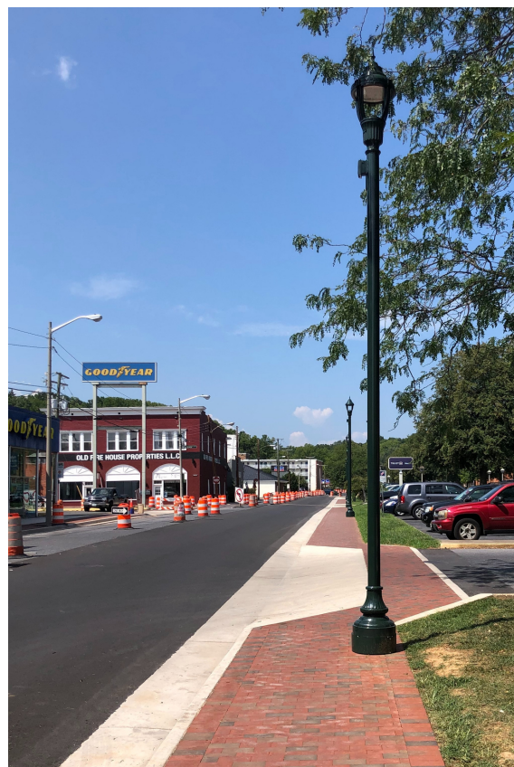
New brick sidewalks, curb, gutter and street lights along Central Avenue
