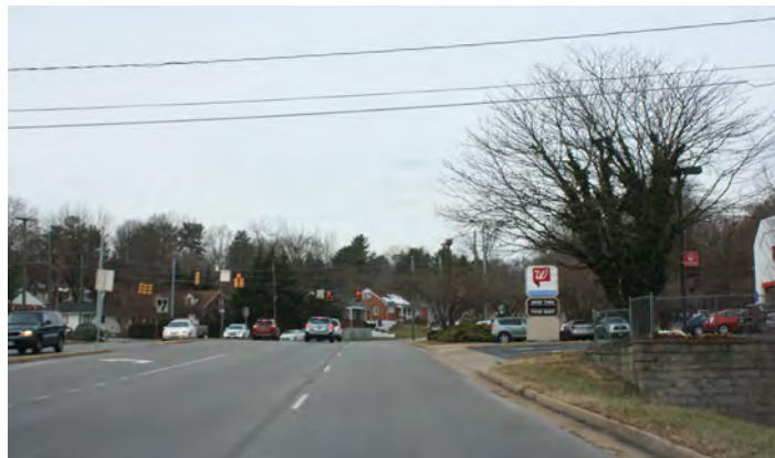
The Coalter Street intersection contains neighborhood commercial uses as the corridor connects to the residential areas of Edgewood Road beyond.
