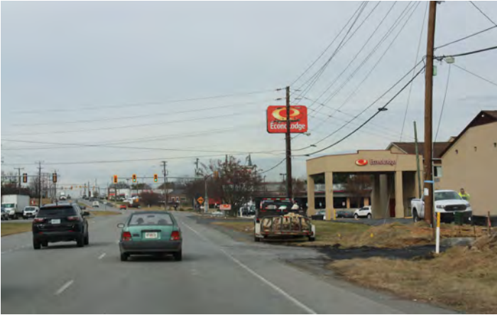
Parts of the corridor lack curb and gutter or sidewalks or any sort of landscaped edge. Overhead utilities abound throughout the route.
