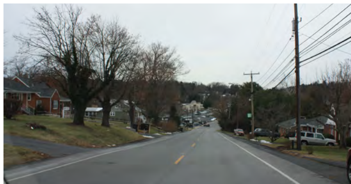
Most of the corridor coming from the north is two lanes with overhead utilities and without sidewalks.
