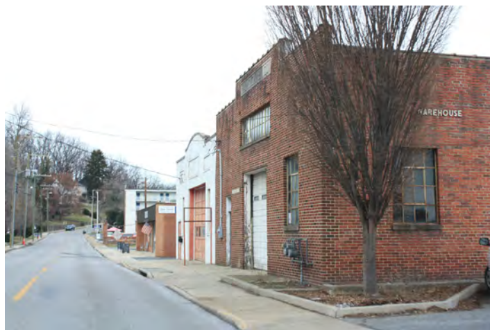
Early 20th century, one-story, industrial service buildings with minimal setbacks still remain on North Lewis Street.
