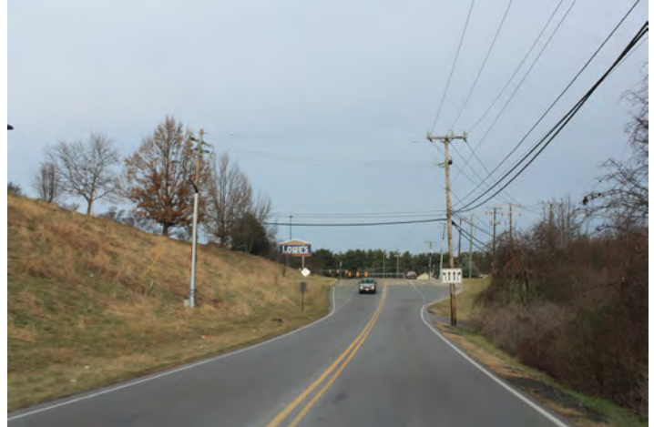
The steep slope of the west side of the corridor still contains a motel and further north access to the Lowe's retail establishment.
