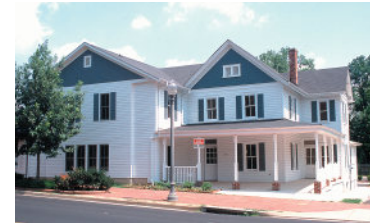
This West Broad Street development converted an older residence to commercial use and added a new wing to it with similar forms and materials.
