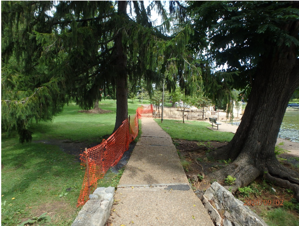
PHOTO 5 - VIEW OF PEDESTRIAN PATH LOOKING NORTH.
