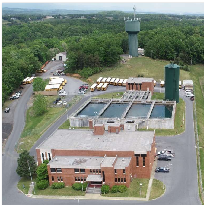
Staunton's Water Treatment Plant
