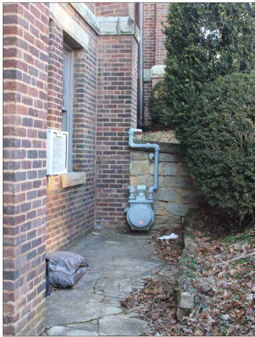
PHOTO: Retaining wall and Gas meter at work area
