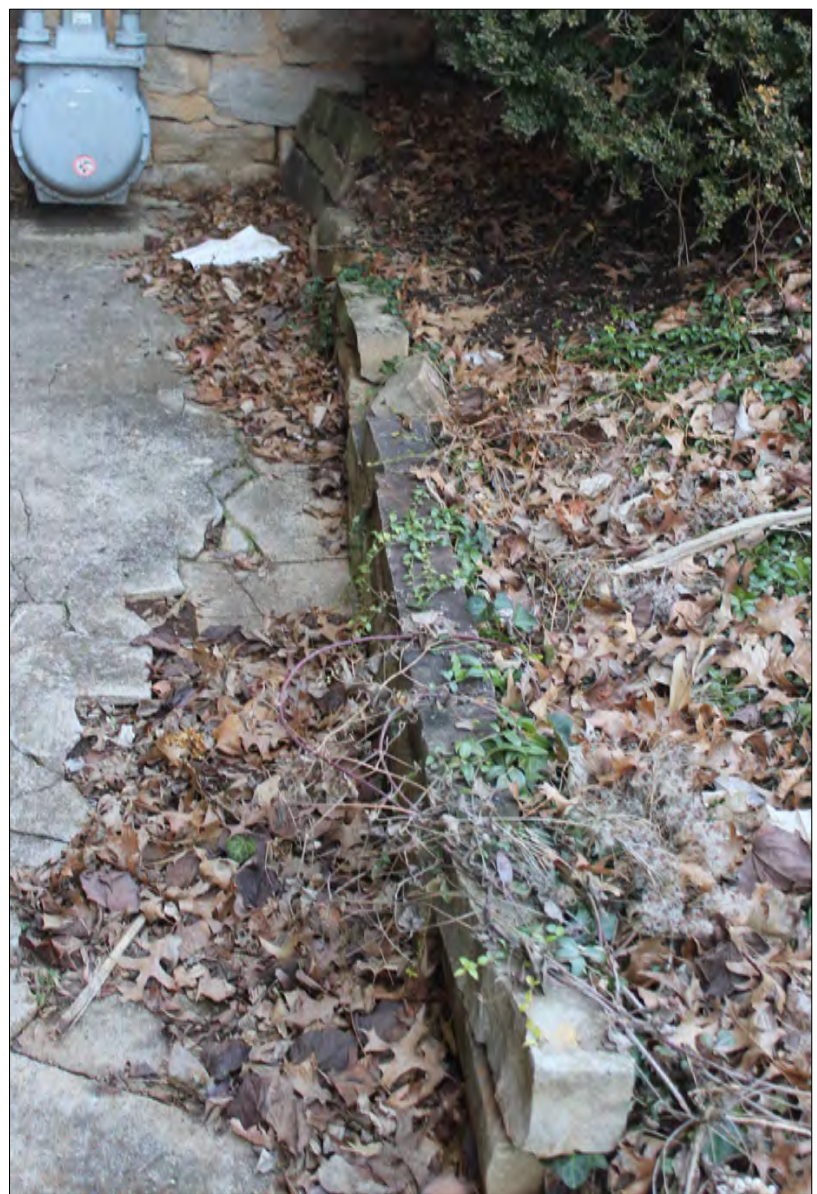
PHOTO: Existing slab/soil edge at work area
