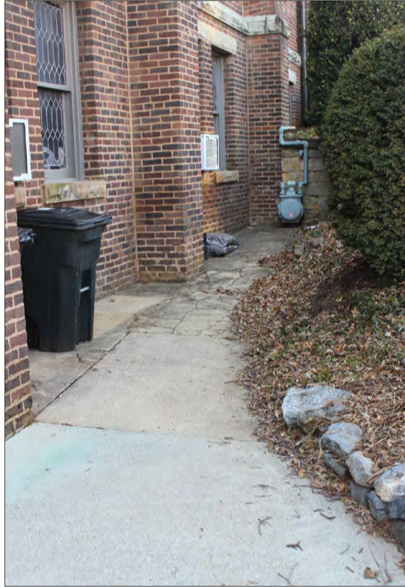
PHOTO: Existing Slab and Gas meter at work area
