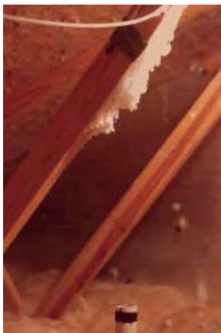
Figure 3. Moist interior air leaking through a hole in the ceiling can produce moldy sheathing or frost on a roof truss. This photo by the author shows results from the Attic Performance Project.
