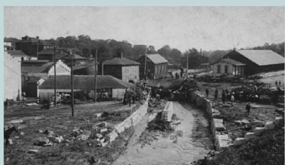
Staunton: 1896 Flood Damage
