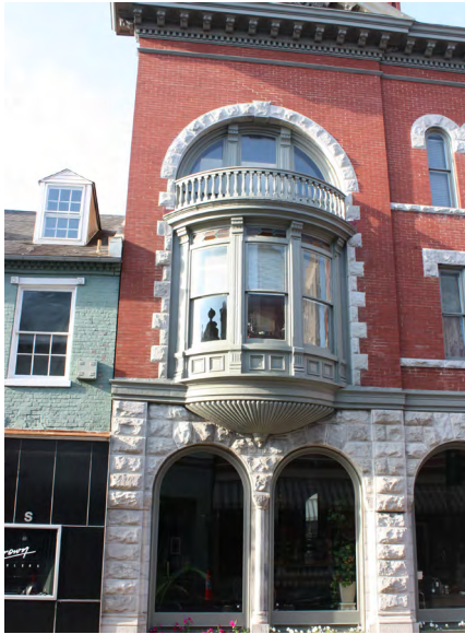
Decorative oriel window with three one-over-one sash & a balcony above in a late 19th c. building.
