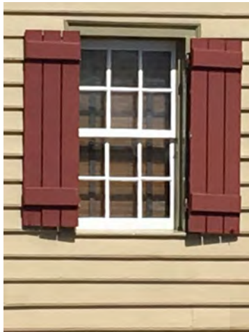
Six-over-six sash in an early 19th c. frame building.
