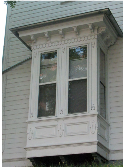
Decorative bay window with double one-over-one sash in a late 19th c. building.
