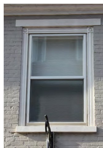
One-over-one replacement sash in a 19th c. brick building.
