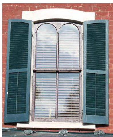
Two-over-two sash in a late 19th c. brick building.
