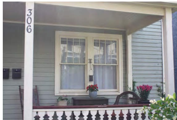
A double window made of two four vertical lights over one sash; this type is seen on early 20th c. buildings including American Foursquare & bungalows.
