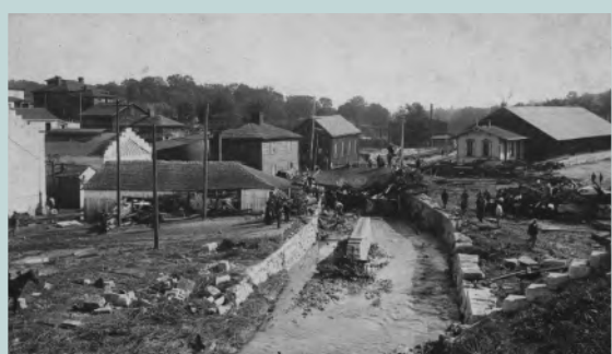
Staunton: 1896 Flood Damage
