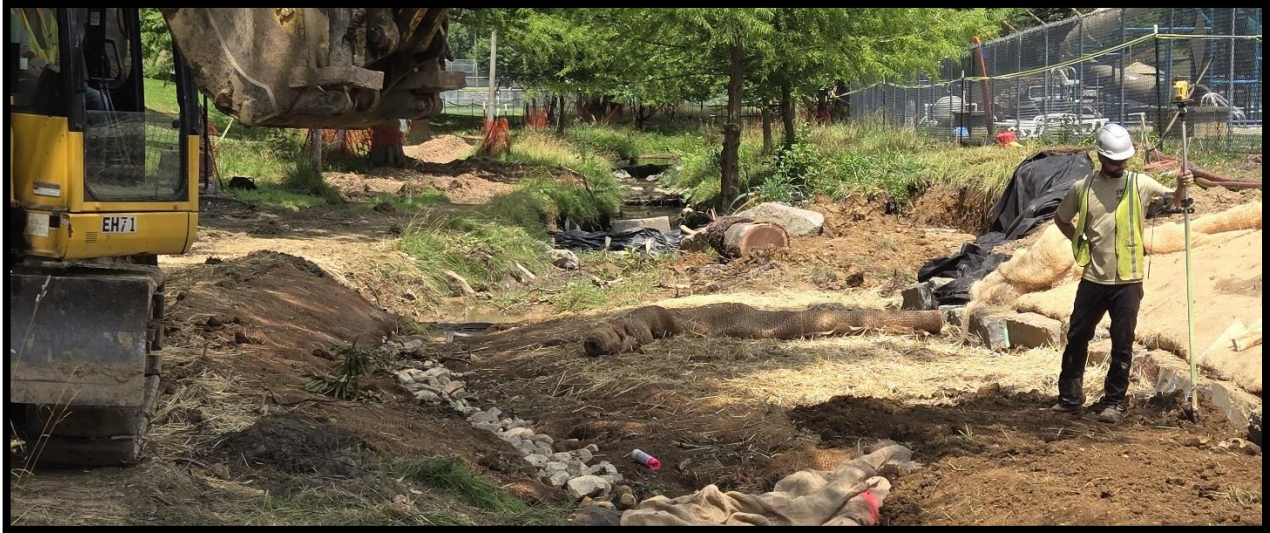
Work continues on the Gypsy Hill Park Stream Restoration Project
