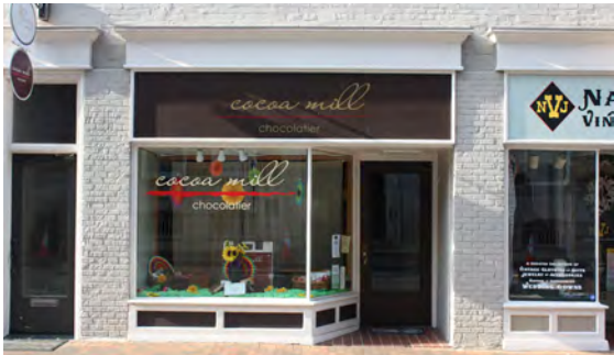
Likely, the interior of these storefronts has a lowered ceiling and therefore the transom became an appropriate location for signage.
