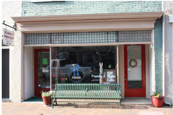
This storefront retains its prism glass tile transom, a rarely surviving feature. Note the door to the upstairs space.
