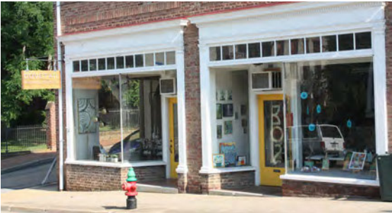
This pair of Colonial Revival styled storefronts retain their original design with the entablatures supported by pilasters. Note the original transom.
