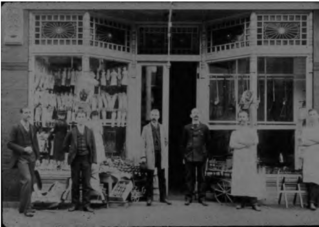
Historic photos often can aid in planning reconstruction of missing storefront elements.
